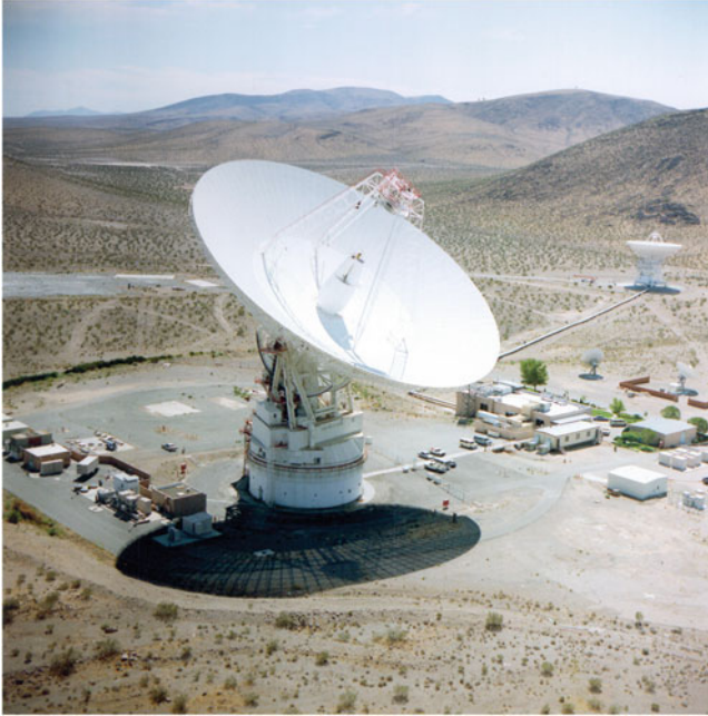
Fig. P.1 Aerial view of Deep Space Network (DSN) at Goldstone, Mojave Desert, Southern California. The giant 70 m dish is in the foreground, a dozen other smaller dishes are located around it spaced up to 10 km's from one another
