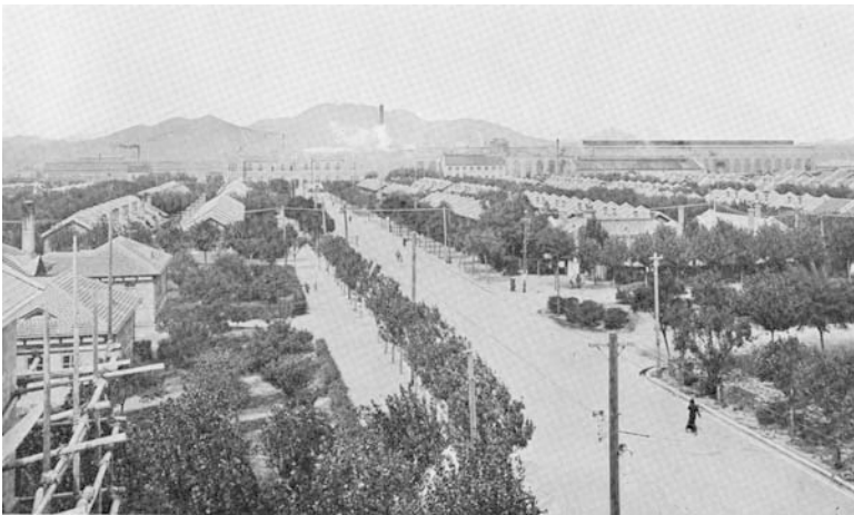
Figure 3.1 View of Fushun, ca. 1920.
