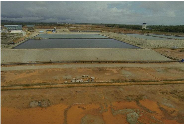
Picture.3. Flooding of the RSF during the monsoon season in December 2013 (courtesy SMSL)
