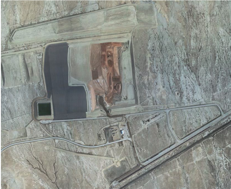
Fig.5. Crescent Junction disposal site, 2014. From left, final cover (dark grey), interim cover placed (light tan), RRM being placed (red), and excavated cell unfilled.
