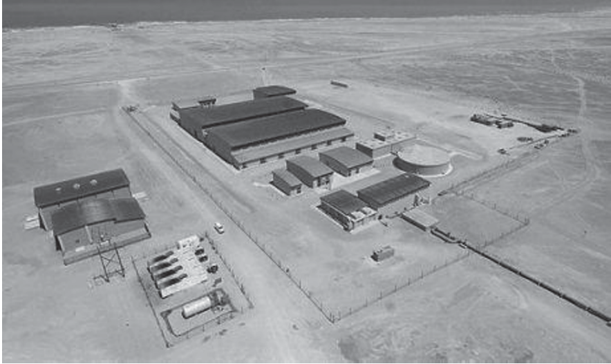
Fig.6. Areva Desalination Plant in Wlotzkasbaken (Source: World Nuclear News 2014).
