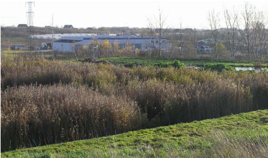
Fig. 8.3 HSSF beds for landfill leachate treatment in Szad?ki, Gda?sk, Poland ( Photo A. Ostojki )
