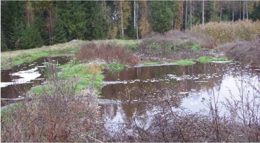
Fig. 8.2 SF wetland for landfill leachate treatment in Atleverket near rebro, Sweden ( Photo Magdalena Gajewska )
