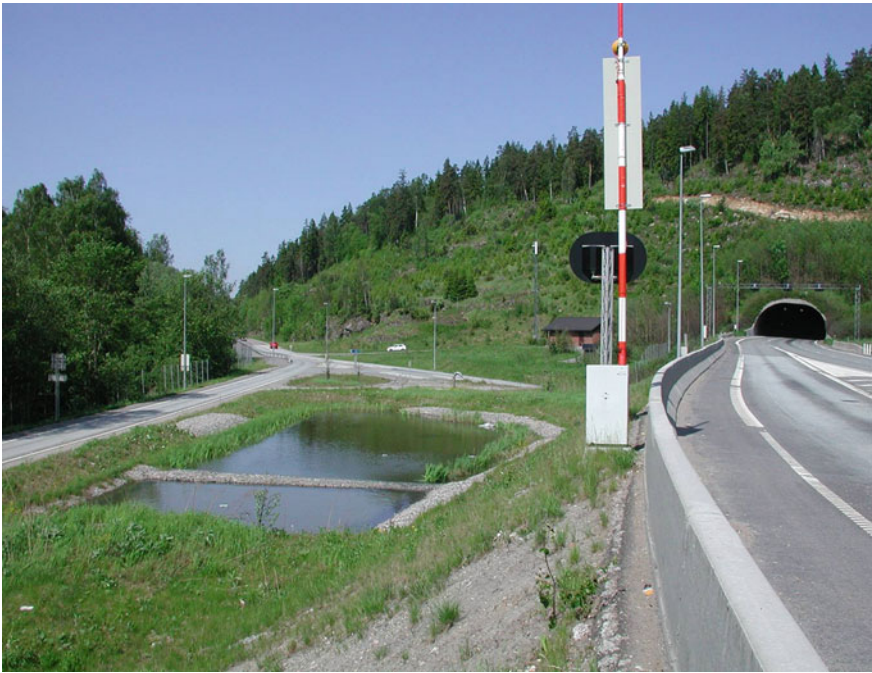
Fig. 6.8 Free water surface wetland for treatment of tunnel and road wash in Norway ( Photo A. Paruch )
