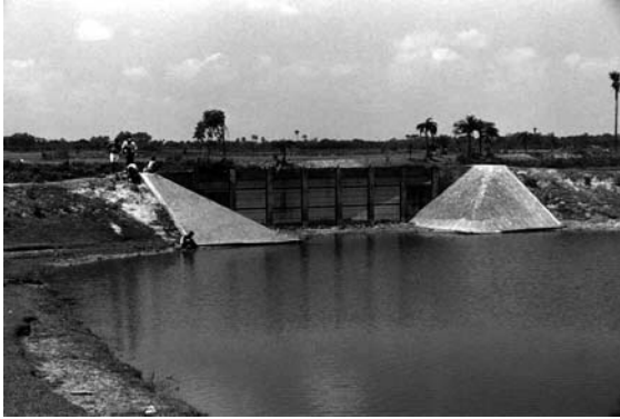
Fig. 8.2 Entrance to floodplain lagoons and poldered areas. A Sluice on inflow canal to an agricultural polder, Bangladesh. B Entrance to a floodplain lagoon complex (fishing lot) with nets to capture fish leaving the lot, Cambodia
