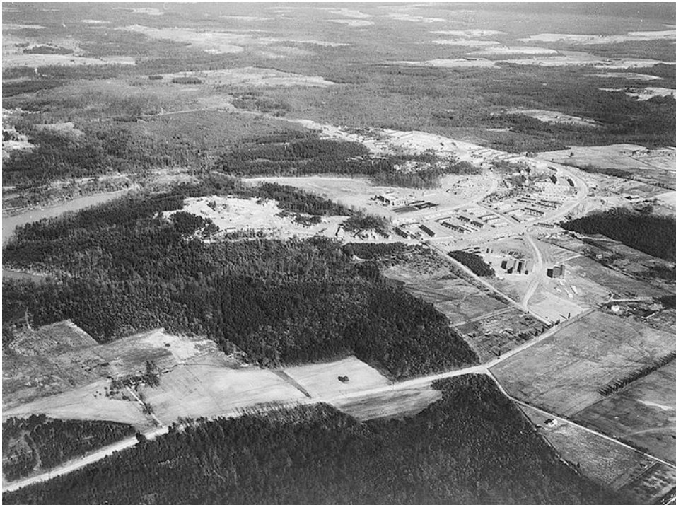
Greenbelt under construction [credit: Farm Security Administration]
