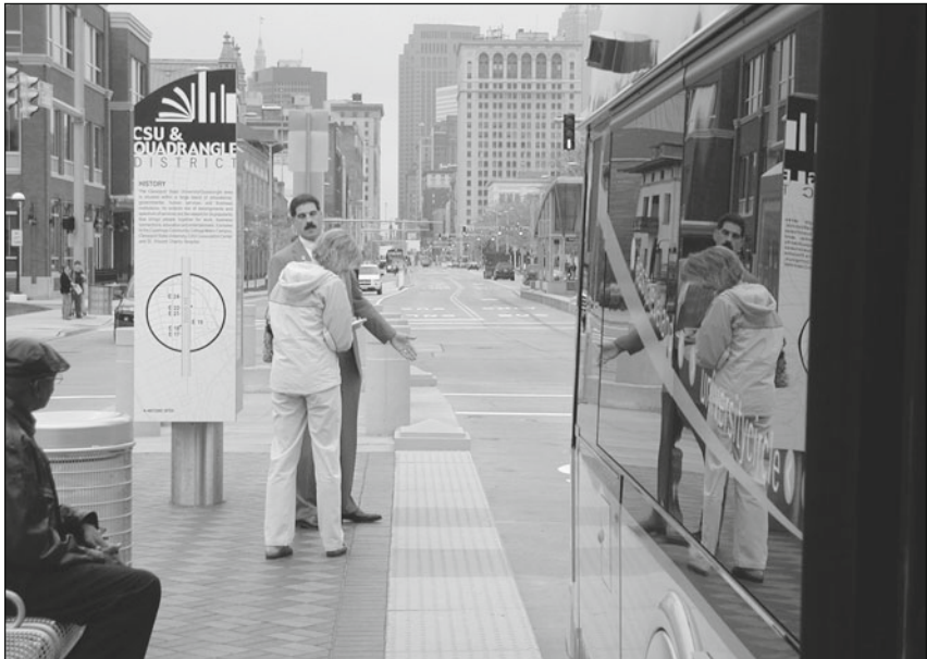
Cleveland's HealthLine reallocated space along Euclid Avenue, dedicating two central lanes to rapid transit, adding transit stations, and narrowing the remaining automobile lanes. (Photo courtesy Jerome Masek/Cleveland RTA.)
