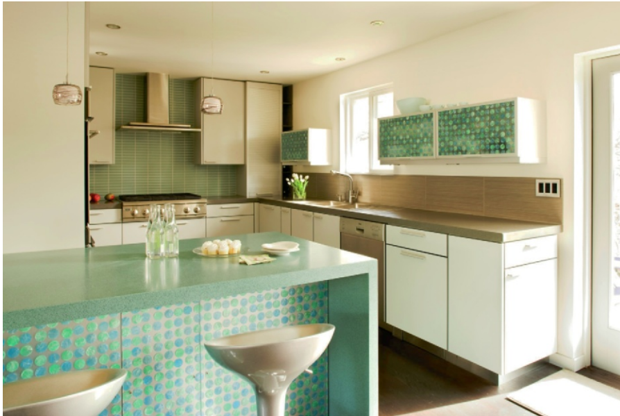
Figure 19.4 The cabinets in this remodeled ranch house kitchen are locally produced and made of wheatboard, a very low VOC and formaldehyde free alternative, with light gray melamine finish. The countertops are Durat, a solid surface material with 35 percent recycled content. The horizontal wall cabinet doors, as well as the back of the peninsula, have panels of 3-form capiz shell ecoresin (with 40 percent recycled content). The backsplash tiles behind the range and the vent hood are unglazed porcelain tiles, also with high recycled content.
