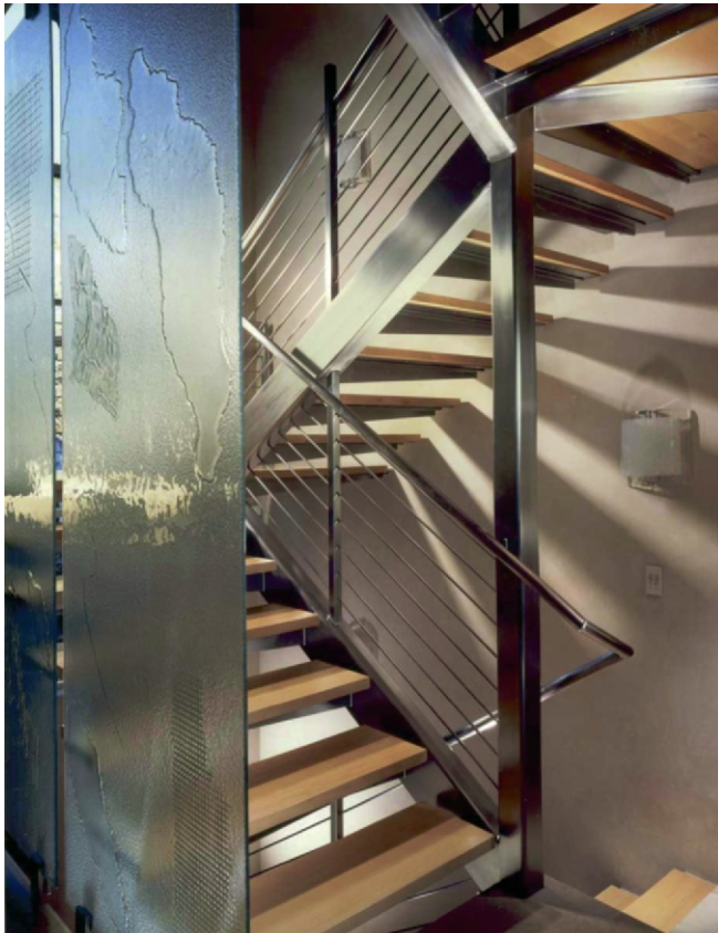
Figure 11.1 Stainless steel staircase railing, stringers, crossbars, and structural-support columns and beams.
