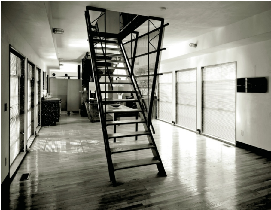
Figure 14.11 This home has recycled oak flooring that was removed from a demolition project in Kansas City, Kansas. This space also features recycled metal stairs and railings and ample daylighting.
