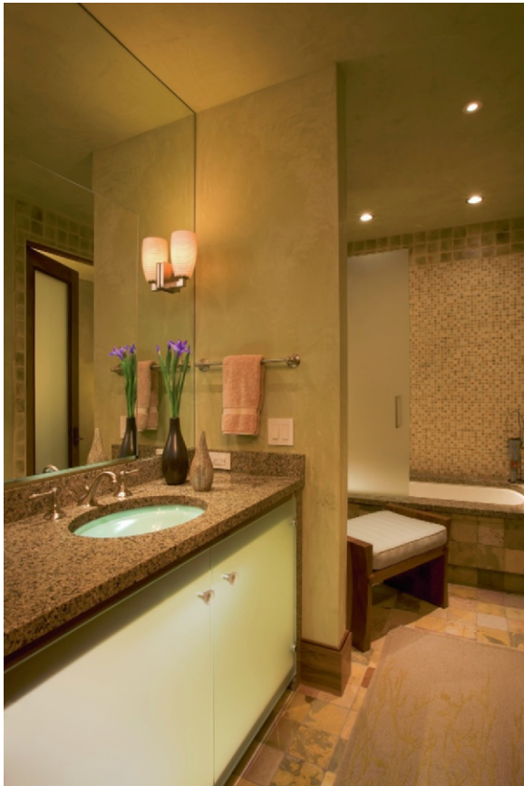
Figure 14.4 This bathroom used integral color earthen plaster on the walls and ceiling. It also features locally crafted recycled glass sink and cabinet doors, Energy Star compact fluorescent lamp (CFL) sconces, recycled content wall tile, and WaterSense plumbing fixtures and fittings.
