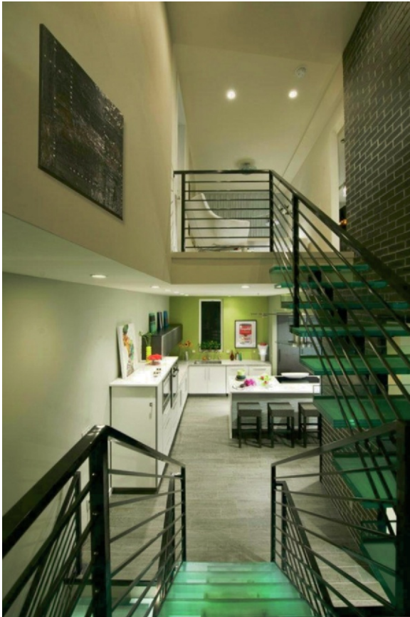
Figure 16.5 The stairs serve as an open, transitional space from the kitchen to the small upstairs home office that makes use of energy-efficient equipment. Also featured is an accent wall created out of Wall Flats made with 100 percent bamboo pulp. Wall Flats are biodegradable and recyclable at the end of their life cycle.
