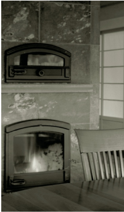
Figure 15.3 This Tulikivi masonry soapstone oven provides heat for the entire home. The space also features solid wood furniture and natural clay plaster.
