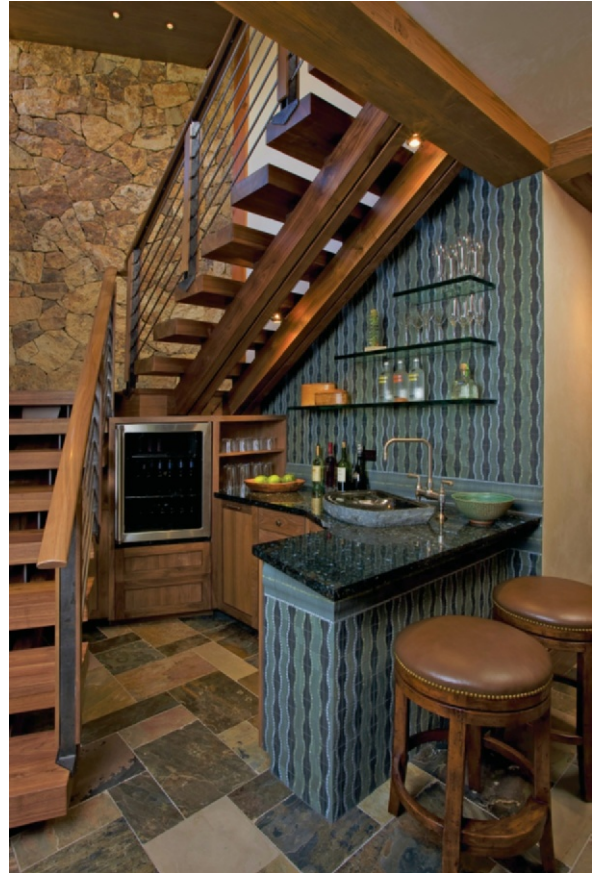
Figure 14.7 This wet bar came from a “found” space under the stairs during a client project walk-through while the home was under construction. The team created a cozy service bar for one with all the requested amenities. The mosaic wall tile is from recycled content glass and stone, used low-VOC installation methods, and features FSC-certified walnut cabinetry and stair treads, slate flooring, and LED lighting.
