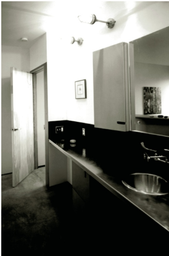
Figure 19.3 This bathroom has a countertop of recycled 1/8-inch aluminum. The space also features natural concrete flooring with integral color and radiant heat, and cabinets made of raw medium-density fiberboard (MDF) with a clear, water-based sealer.
