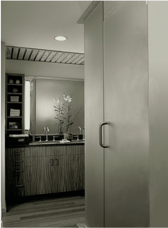
Figure 15.2 This bathroom has a shower door of frosted, frameless glass. The space also features a green slate countertop, recycled glass tile in the shower, anigre wood cabinetry, a wood ceiling from a reforested area, fluorescent lighting, and low-VOC paint.
