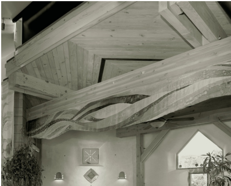
Figure 12.2 This handcrafted millwork was made from trees on the site that were killed by a fire.
