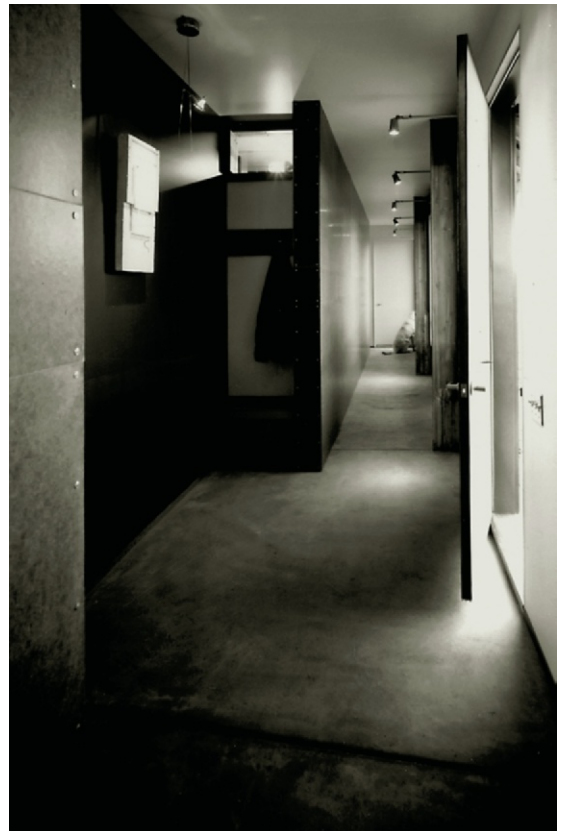
Figure 9.3 This gallery has radiant-heated concrete floors with a natural color pigment added and has been sealed with linseed oil. The space also features recycled-content Masonite walls with integral color added, also sealed with linseed oil.
