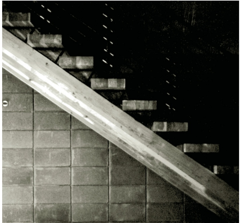
Figure 12.6 The treads and stringer of this staircase were made from pine glulams, which were assembled by gluing smaller pieces of wood together, thereby avoiding the need to cut down old-growth trees.
