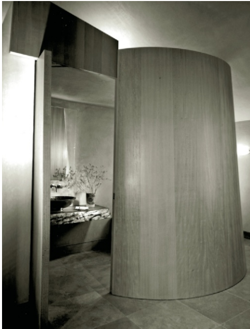
Figure 13.2 A locally crafted pivot door and curved wall of sustainably certified beech enhance the entry to this powder room.
