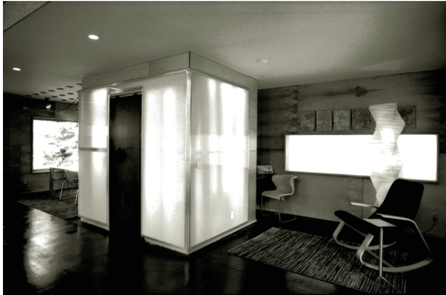
Figure 18.3 This powder room cube features fluorescent lighting inside the walls. The space also features a 50 percent recycled content steel door and fiberboard walls.
