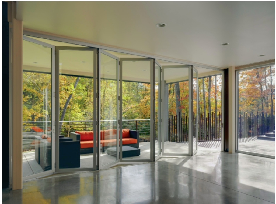
Figure 13.4 The Zinc House features LaCantina Doors' contemporary aluminum folding door system. The seven-panel operable glass wall spans nearly 23 feet in width.
