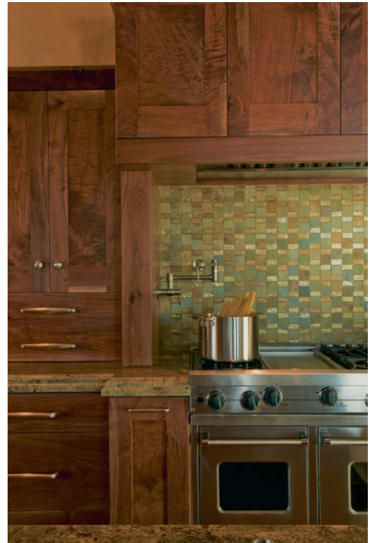
Figure 12.3 Reclaimed wood cabinets were crafted from rescued black walnut trees that had been blown down in a storm. The interior cabinet box is made from furniture board with no added urea-formaldehyde, and water-based glues were used to fasten the wood together and attach the veneer. The finish is a water-based, low-VOC material that lets the wood's beautiful natural color shine through.
