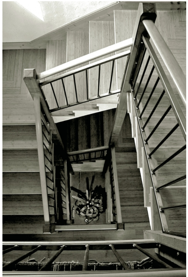
Figure 14.9 This stairwell is constructed of bamboo stair treads, risers, and nosings. This space also features a railing made from unpainted steel with a low-VOC clear sealer and walls finished with no paint “tinted gypsum plaster.”
