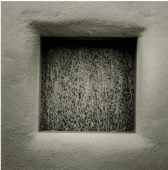
Figure 21.1 This truth window offers insight into a strawbale wall.
