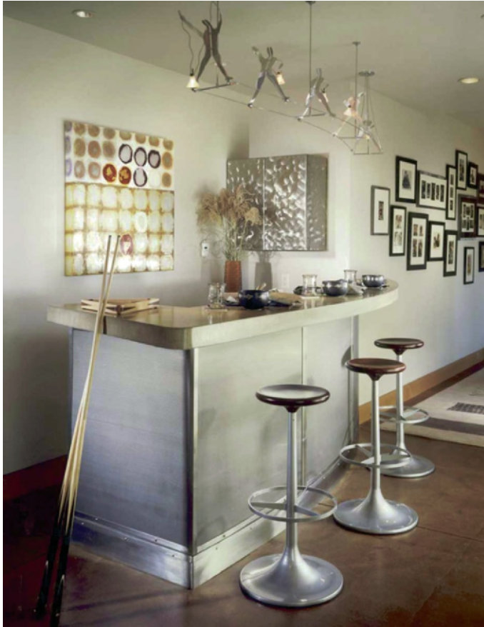
Figure 9.1 A graceful, locally manufactured concrete countertop and concrete slab stained floor. The photo also captures recycled steel bar framework and cabinet, LED lights, and zero-VOC paints.
