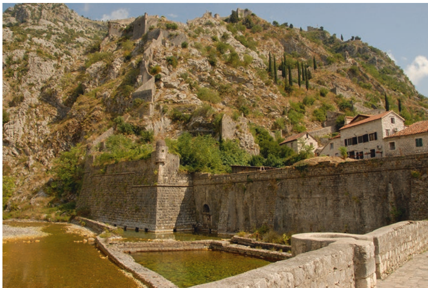
Fig. 3.11 The northern walls of Cattaro ( photo by PA, 2011)
