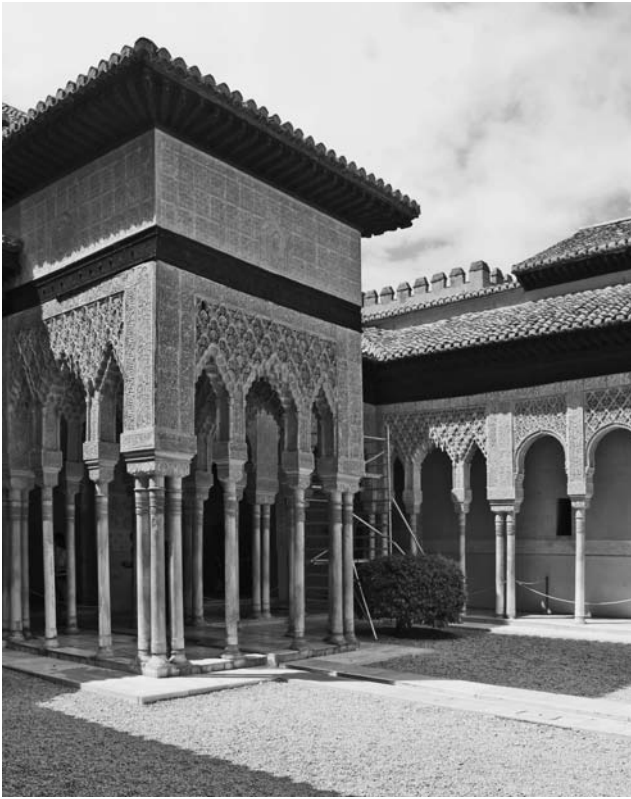
Figure 5.42 Alhambra. The eastern pavilion of the Palacio de los Leones.
