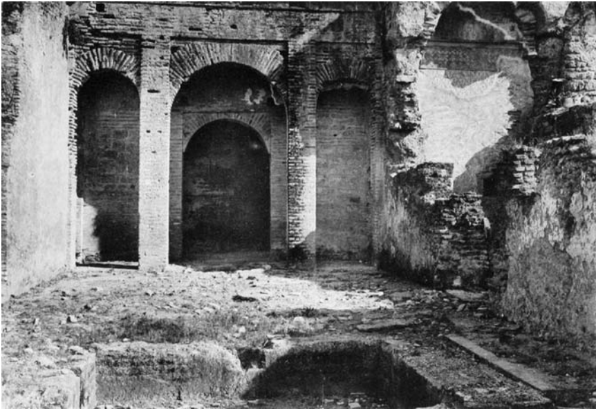
Figure 5.3 Tlemcen. Main courtyard of the palace at al-Ubbād.
