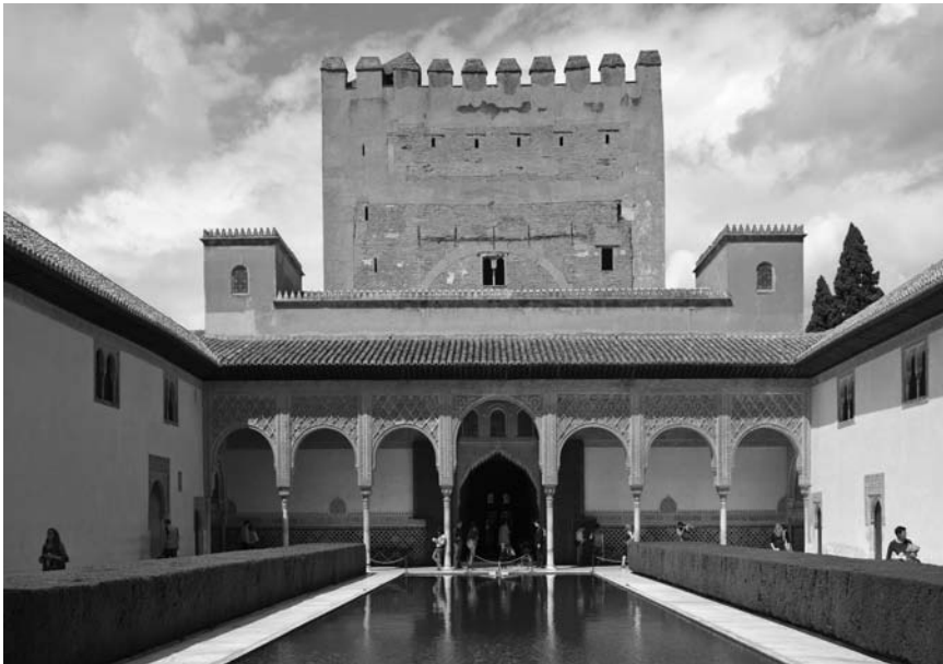
Figure 5.31 Alhambra. The courtyard of the Palacio de Comares.
