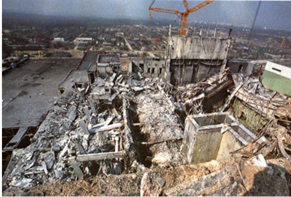
Fig. 8.3 Chernobyl #4 reactor accident
