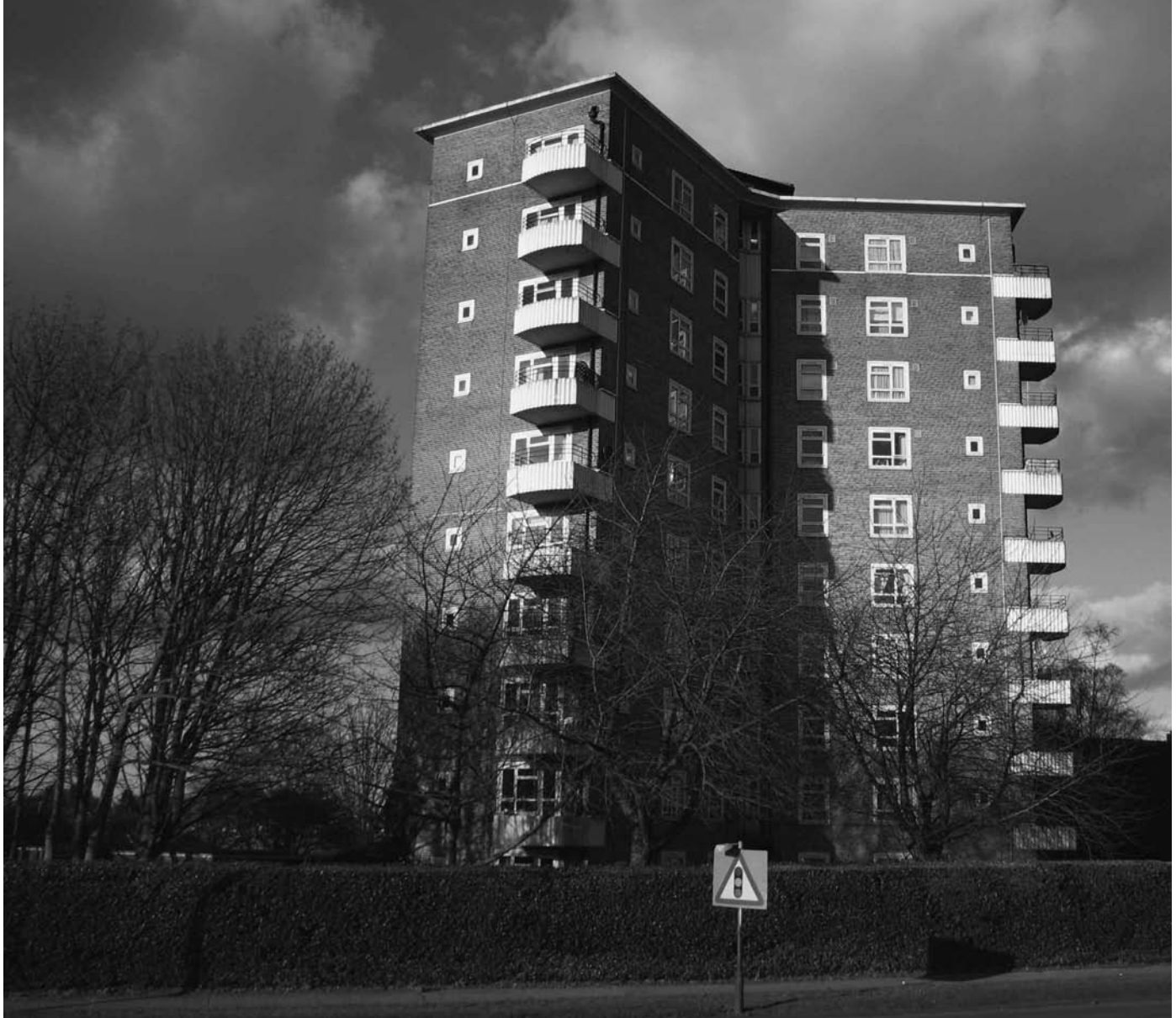
Gibberd's eight-storey block, The Lawn in 1951, was Britain's first towerblock.
