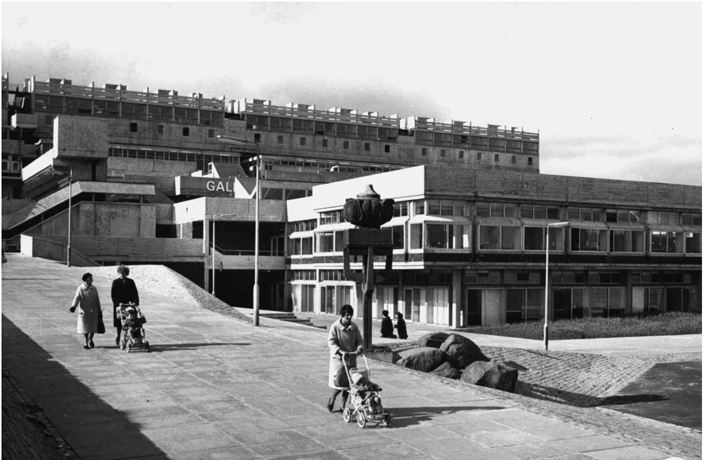
Cumbernauld's centre was built on top of a steep hill. Copyright: North Lanarkshire District Council.
