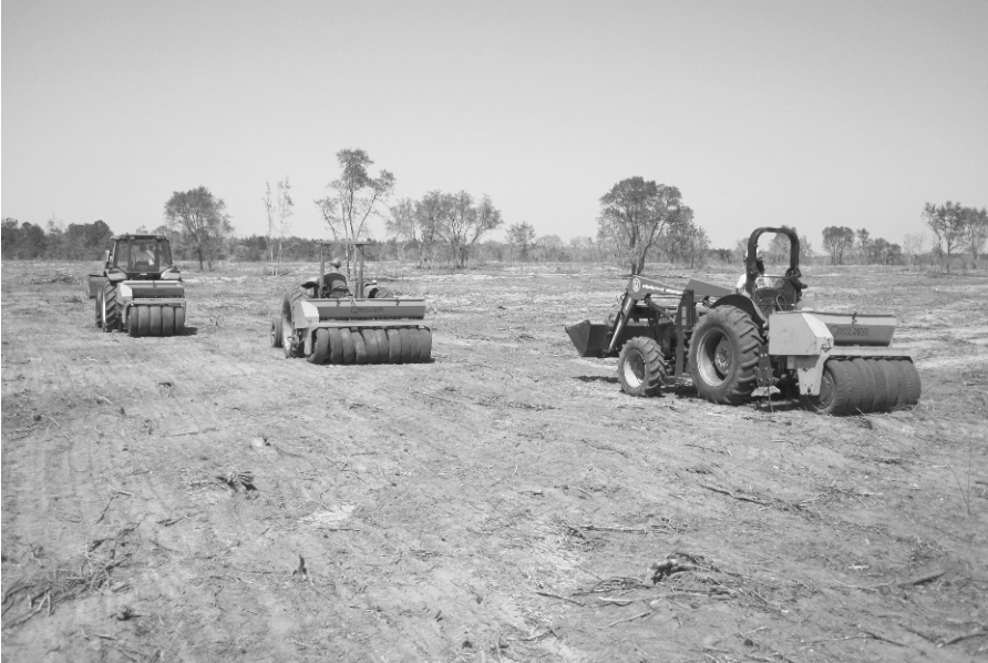
PHOTO 3. Three, tractor-drawn Grassland® planters planting undergrowth seed mix on a newly prepared project site.
