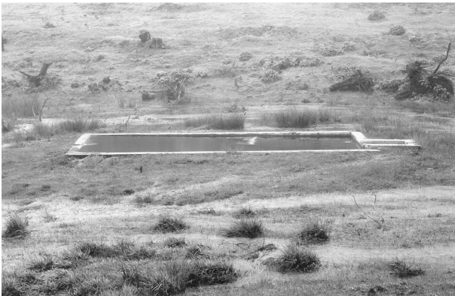
PHOTO 2. Pool excavated in dried-out marsh to provide water for wildlife.
