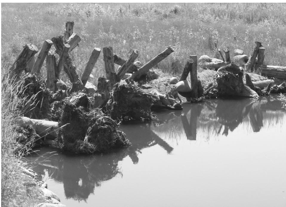
FIGURE 5.3. Large woody debris used in stream restoration both as armament to redirect flows and stabilize banks, and as habitat for macroinvertebrates and fish, in the Olympic Peninsula of Washington state, USA.
