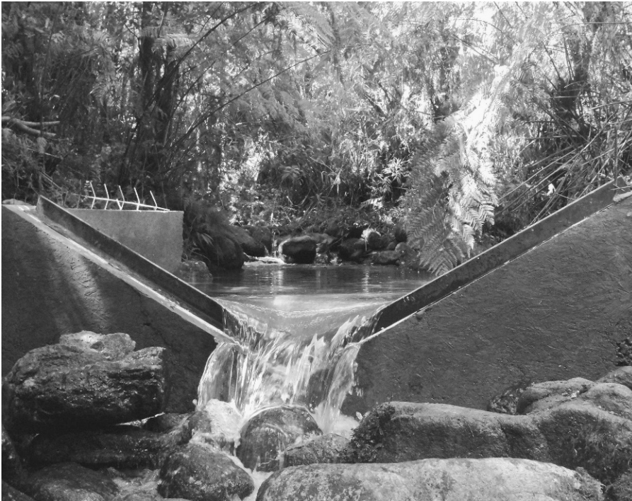
Photo 6. V-notch weir in a stream to measure water yield.
