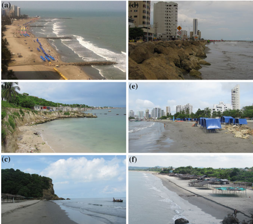
Fig. 3.2 Major geomorphologic characteristics observed along Cartagena area (Colombia). Groins along Bocagrande Beach (a), cliff erosion at Tierrabomba island (b), beach and cliff at Los Morros (c), rip-rap revetment at Crespo (d), tourist area at Castillogrande (e) and beach escarpment along Los Morros (f)
