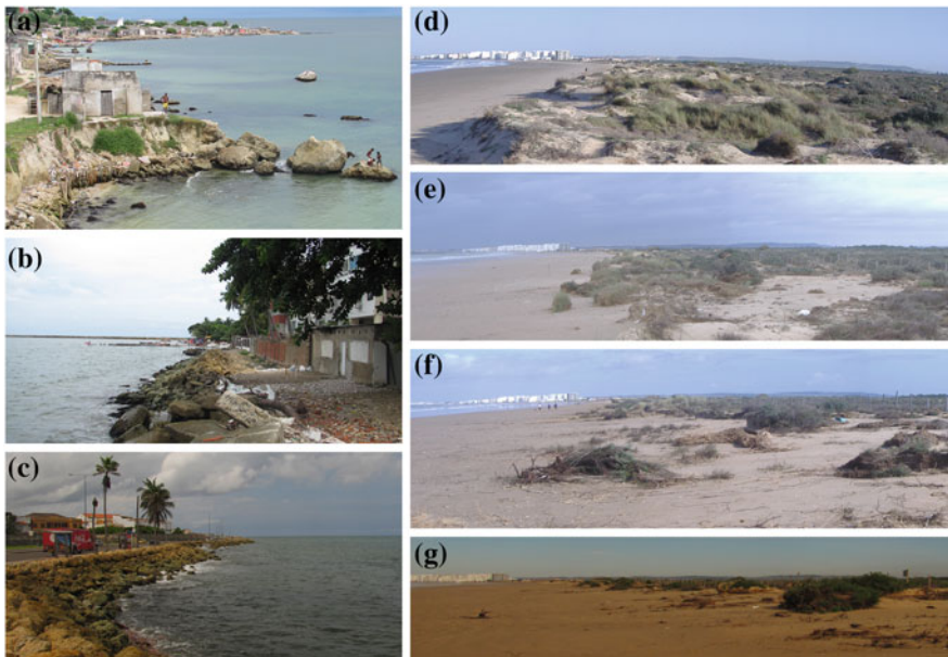
Fig. 5.4 Examples of coastal erosion along Cartagena and Cadiz areas. Cliff erosion at Tierrabomba (a), erosion and rip-rap revetment at Bocagrande (b) and Marbella (c) beaches, sequence of coastal erosion at Valdelagrana beach, 16-11-2009 (d), 06-01-2010 (e), 12-03-2010 (f), and 24-12-2010 (g)
