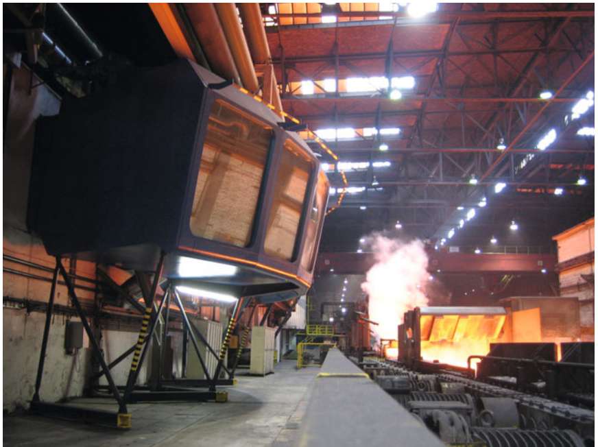
Visitors' platform overlooking the hot rolling mill, caramel architekten, Friedrich Stiper, 2006. Photo: Ulrich Aspetsberger.
