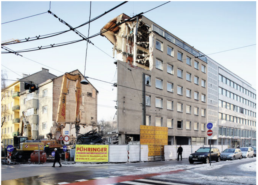
2010 demolition of the Community College, former Park Hotel, constructed in 1952 by Artur Perotti and Gottfried Zellingner. Photo: Gregor Graf.
