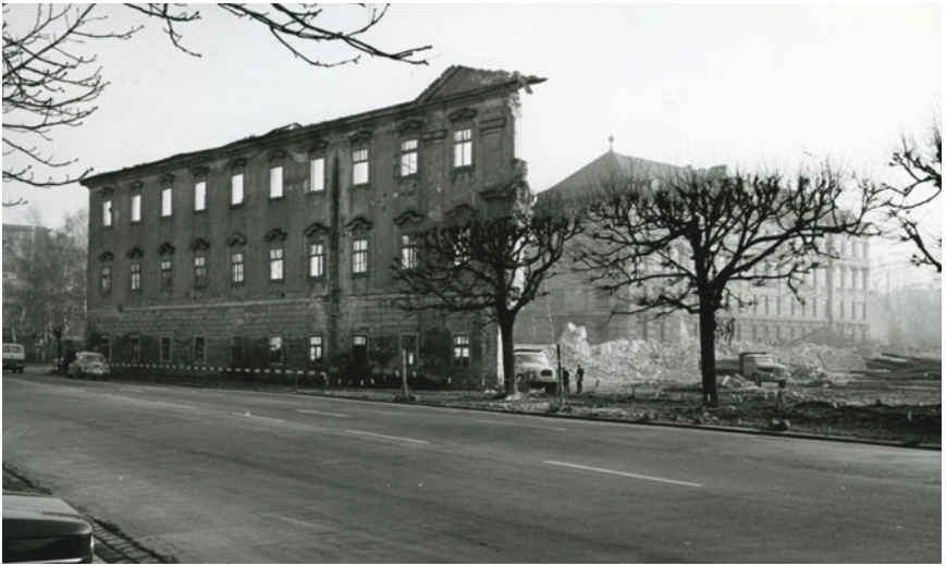
Demolition of the Wool Factory, 1969. Photo: Archives of the Nordico City Museum, Linz.
