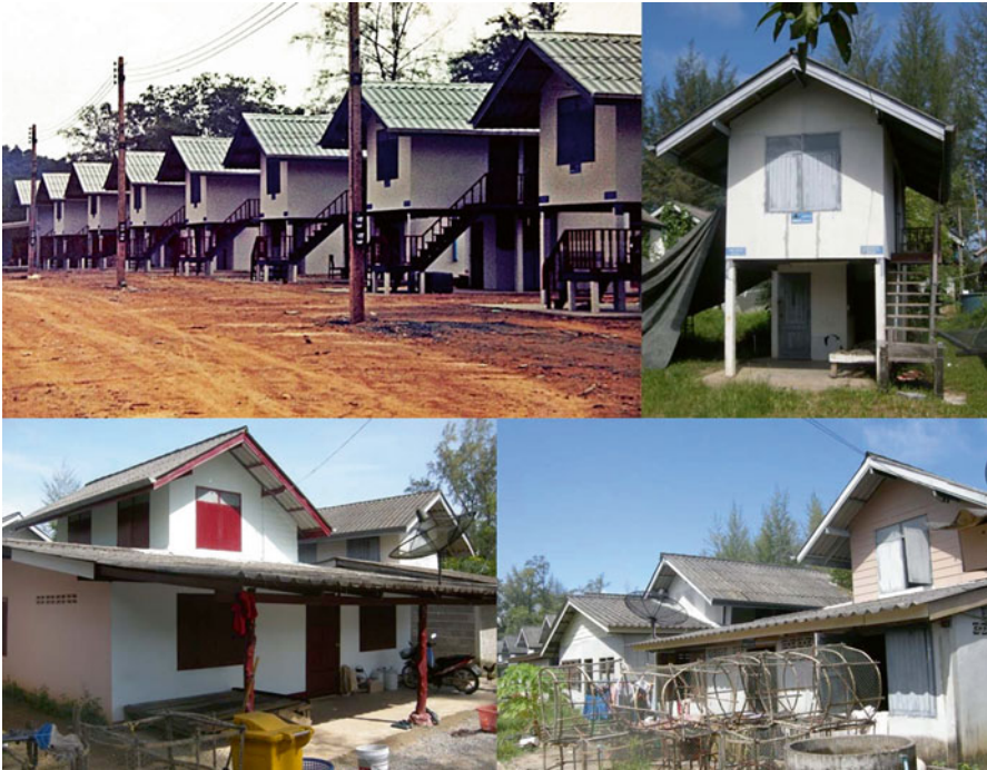
Fig. 6.9 The (then) newly built tsunami resilient houses at Nua village: at the beginning after the construction completed ( top left : photo taken late 2005-early 2006, image by the Tambon Kamphuan Community Learning Center), house waiting to be renovated ( top right , photo taken in August 2013) and the renovated houses ( bottom : photos taken in August 2013)
