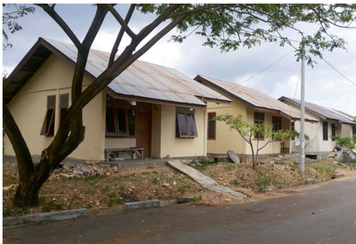
Fig. 5.3 Permanent house built by MDF in the village of Lambung
