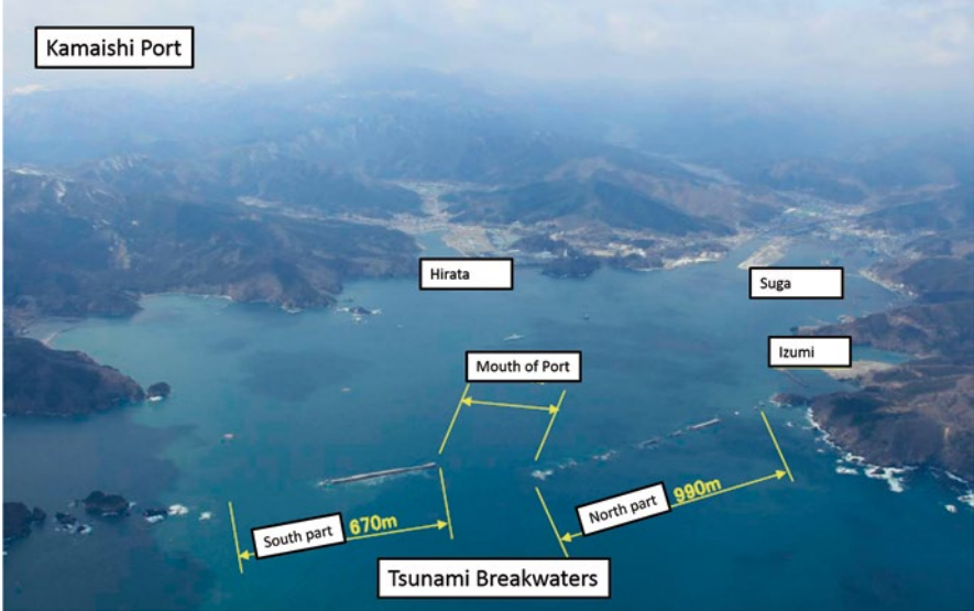
Fig. 14.1 View of the Breakwaters at the Mouth of Kamaishi Port after the 2011 Tsunami (Source: Tohoku Regional Development Bureau; Japan)
