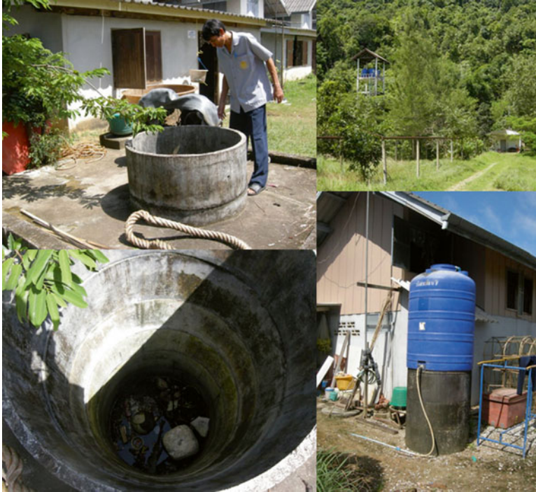
Fig. 6.11 A shallow water wells at the Nua village ( top left photo). Many wells are abandoned due to intrusion of the brackish water, especially during the dry season ( lower left photo). The new water storage tank was constructed at the higher elevation nearby ( top right photo) which released the water to the village occasionally. The released water was then kept in a storage tank at the individual house ( lower right photo)
