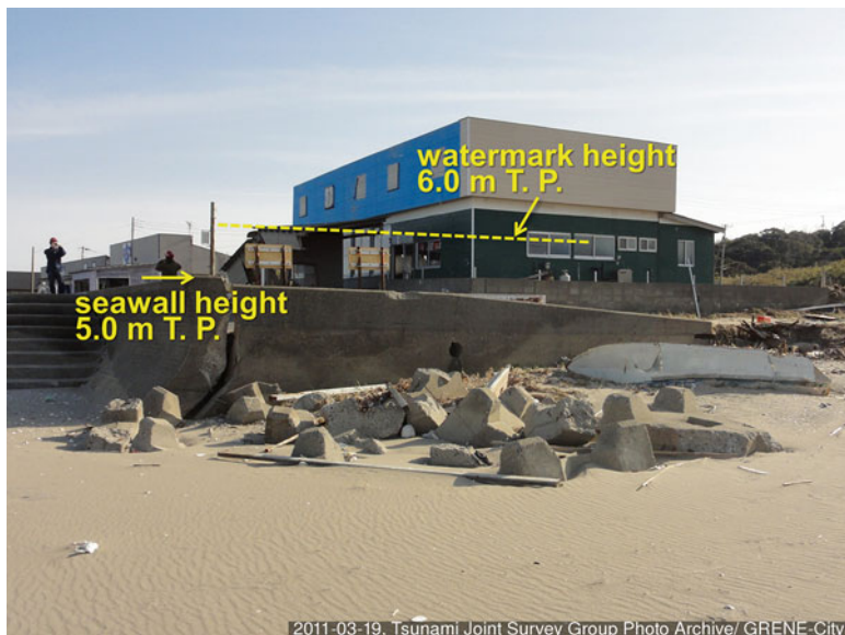
Fig. 13.4 Tsunami watermark measured in Hokota, Ibaraki Prefecture (March 19, 2011); watermark measured at 6.0 m T. P., 55 m from the shoreline (UTMS-0181 in the TTSG database, location marked in Fig. 13.2)
