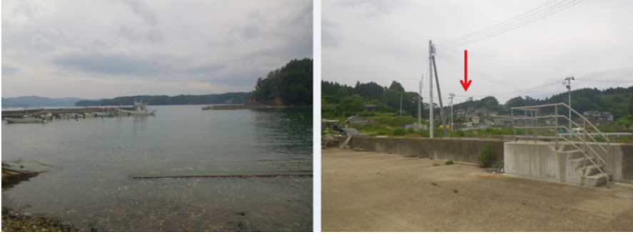
Fig. 4.5 Left : A fishing port is submerged during high tide, but some aquaculture activities were observed ( left ). View of evacuation shelters located behind the high ground from the fishing port ( right ) (Source: Cabinet Office, Government of Japan)
