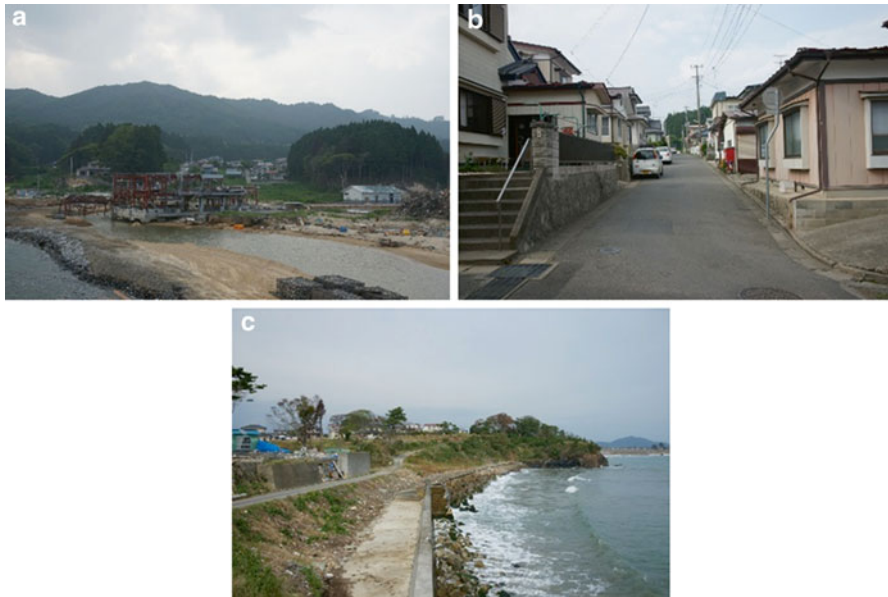
Photo 1.1 Meiji resettled community; (a) Funakoshi, no residential use in low land, (b) Funakoshi community after the EJED; (c) Ootani community (Source: Miyagi Prefectural Government)
