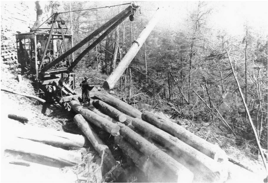
Figure 3.3 Champion Fibre skidder in North Carolina, ca. 1918. Lumber companies like Champion used steam-powered cables to pull logs through the forest to waiting trains. Mechanization increased logging efficiency but damaged the forest floor. Archives, Great Smoky Mountains National Park.
