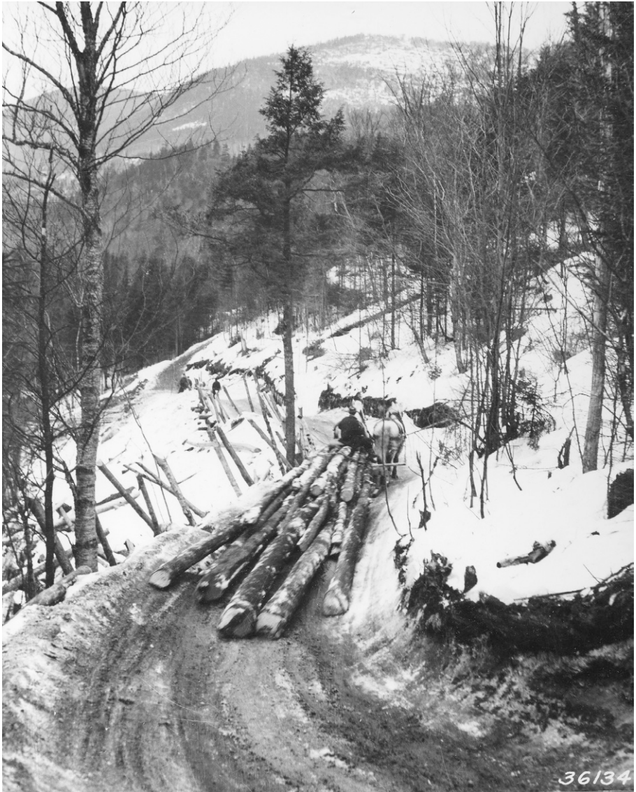
Figure 1.1 Logging road in Lincoln, New Hampshire. During the nineteenth and early twentieth centuries in the White Mountains, loggers used horses to haul logs along dirt roads, causing considerable erosion. USDA Forest Service, Eastern Region Photo Archives.
