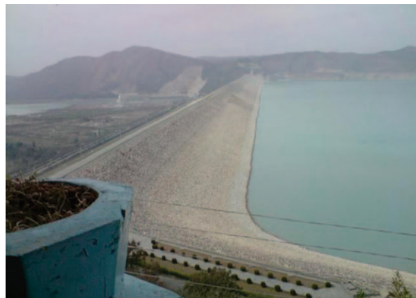
Fig. 12 Tarbela dam -general view
