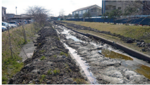
Fig. 29 Upheaval of the river bottom in Jukken Brook, Sawara, Katori—A view to the west from point A in Fig. 25 (from Katori city office)
