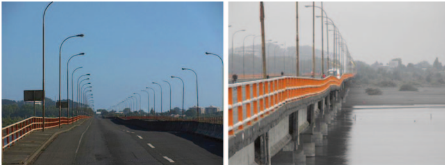
Fig. 21 Settlements along Juan Pablo II Bridge with no evidence of horizontal displacements
