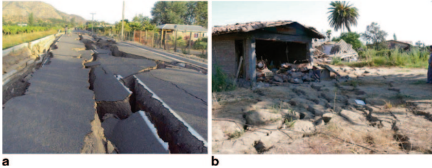
Fig. 16 Lateral spreading observed in. a Apalta route and. b Nancagua Town
