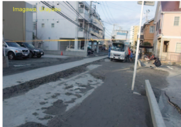
Fig. 21 Thrust of an alley in the Imagawa district of Urayasu City
