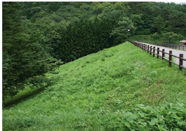
Fig. 29 Pre-earthquake photograph of crest and downstream slope of Fujinuma Main Dam
