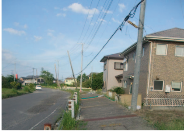
Fig. 15 Tilting of houses accompanied by settlements at Hinode, Itako
