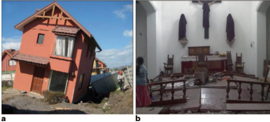
Fig. 13 a Liquefaction-induced failure in Talcahuano, b Church located in Abrantes
