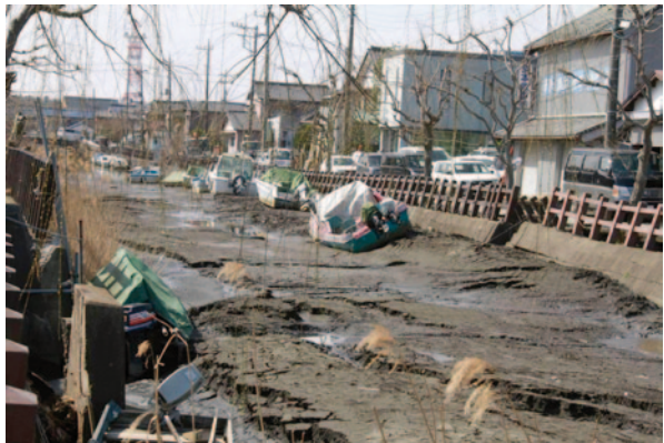
Fig. 28 Devastation in the downstream reach of the Ono River (from Katori city office)
