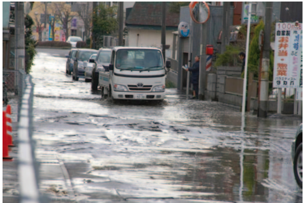
Fig. 27 Flooding of liquefied soils over the road in Sawara, Katori (from Katori city office)
