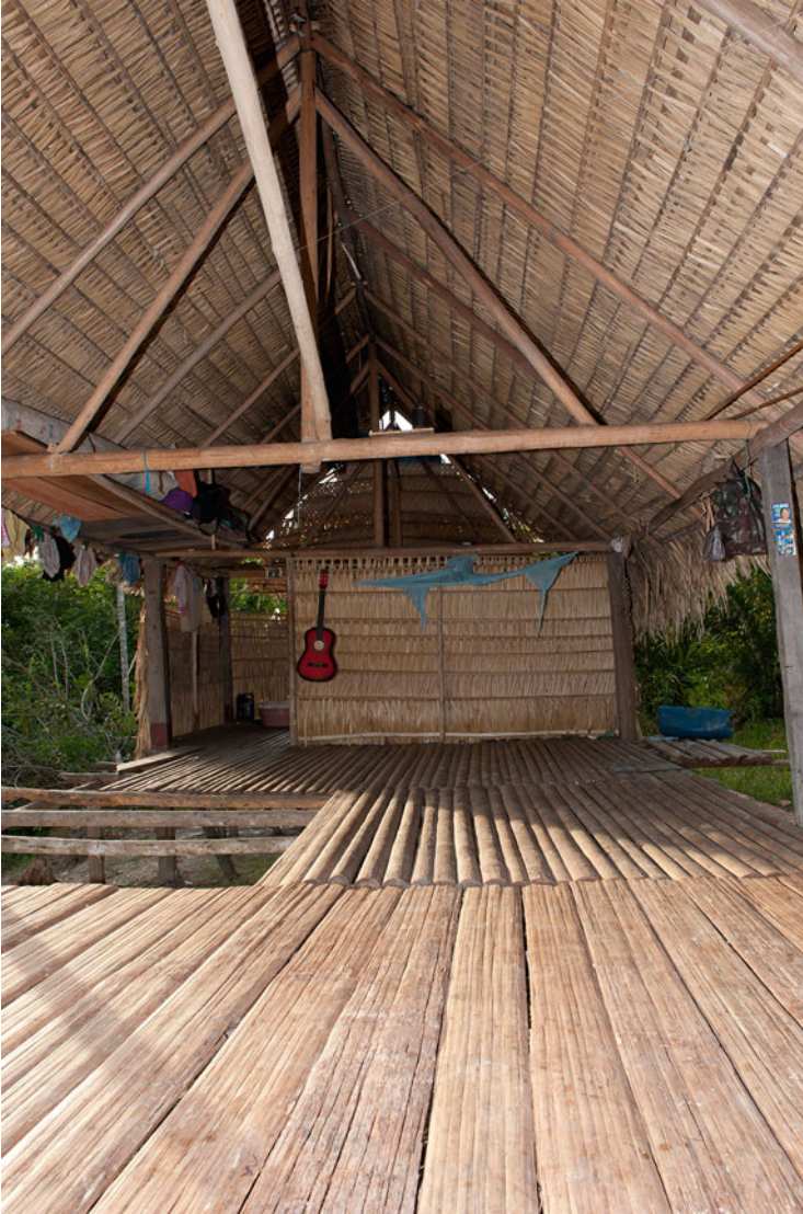
Fig. 35.10 Floor of river dweller's home consisting of split trunks of açai ( Euterpe precatoria ). Palha branca ( Attalea speciosa ) fronds have been used for thatch. Near Seringalzinho, Jaú River, Amazonas, Brazil, 10-3-12
