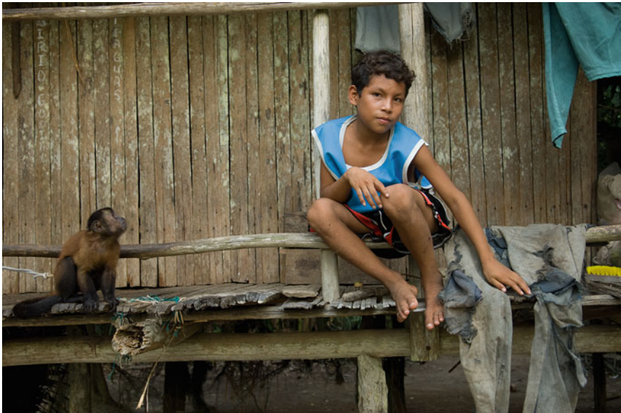
Fig. 35.9 Village house with walls made from split trunks of chonta ( Euterpe precatoria ). The floor is fashioned from split trunks of cashapona ( Socratea exorrhiza ) palm. Yarina, Yanayacu River, Pacaya-Samiria, Loreto, Peru, 1-15-06
