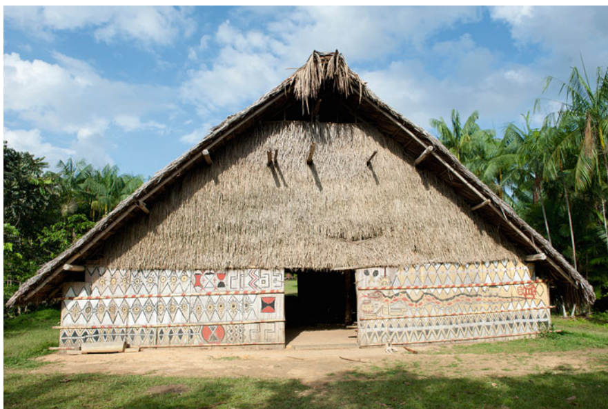
Fig. 46.6 A Tuyuka maloca thatched with caraná fronds. Fronds of açai ( Euterpe oleracea ) cover each end of the communal center above the doorways. São Pedro, Tiquié River, Amazonas, Brazil, 11-2-12
