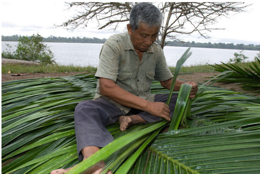
Fig. 14.7 A 72 year-old river dweller fashioning a cumba with fronds of Attalea phalerata in front of his village home. The cumba will be used to repair the roof of his house. San Martin Tipishca, Samiria River, Pacaya-Samiria, Loreto, Peru, 7-16-10
