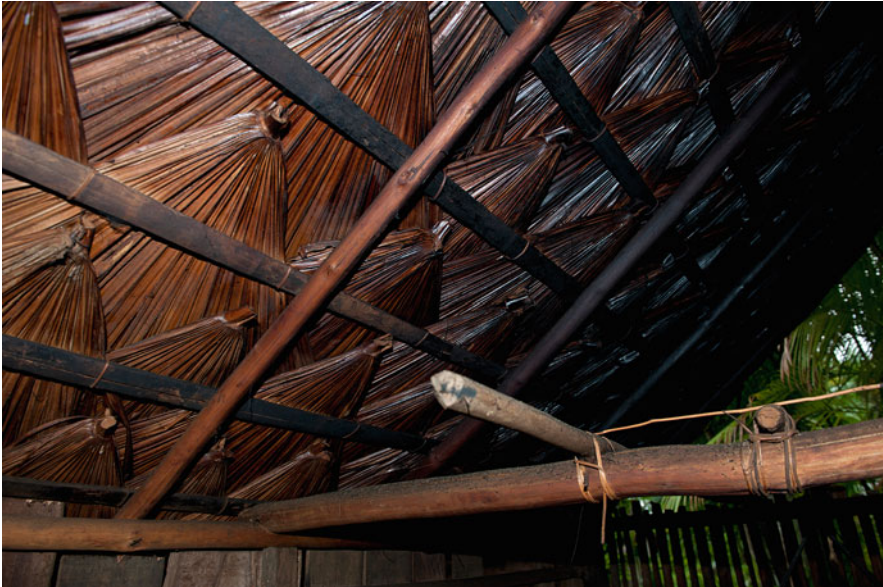
Fig. 46.7 Caraná thatch blackened from smoke from a cooking fire in an external kitchen. Ilha de Taraqua, upstream from São Gabriel da Cachoeira, Rio Negro, Amazonas, Brazil, 10-26-12
