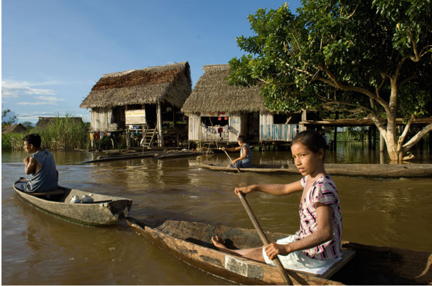
Fig. 44.5 The thatch on the house on the left has been partially repaired with irapay, easily distinguished by the band of copper-colored fronds. Miraflores, confluence of the Tigre and Marañón Rivers, Loreto, Peru, 4-26-06
