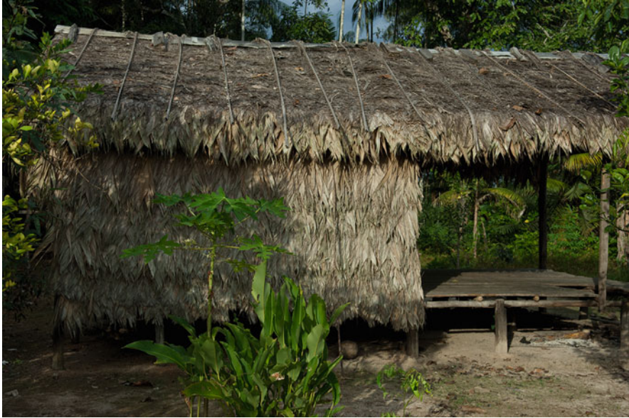
Fig. 36.2 Farm house with roof and walls of Geonoma deversa fronds. Igarapé Açu near Anori, Amazonas, Brazil, 6-22-07
