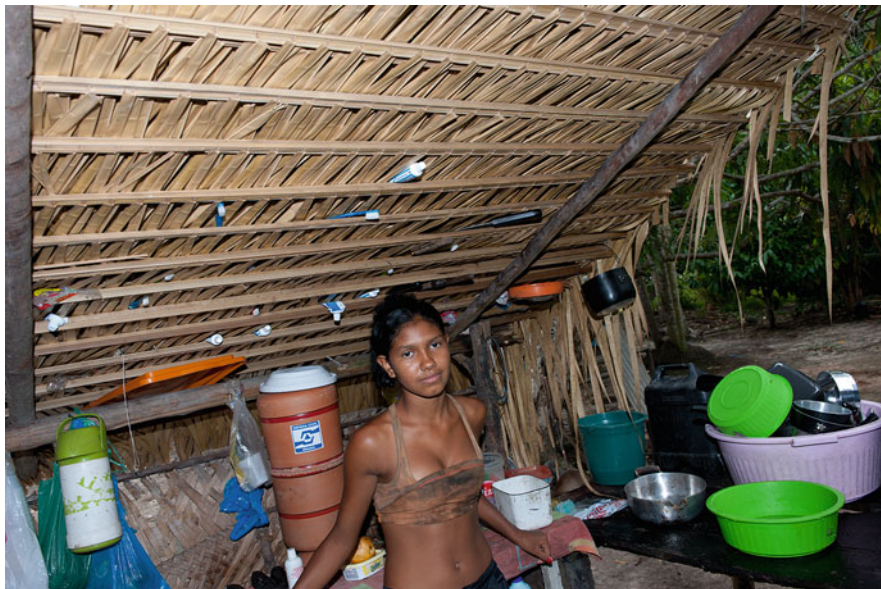
Fig. 15.2 Kitchen in a village home with walls and roof made with Attalea racemosa fronds. Known locally as curuá, the fronds were gathered in nearby upland forest. Sítio São Cristovam, Rio Negro near its confluence with the Jaú, Amazonas, Brazil, 10-4-12
