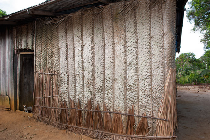
Fig. 16.3 Tukano house the outside wall composed of woven fronds of Attalea sagotii . The base of the wall has fronds of Mauritia flexuosa tucked under a lattice to act as a splash guard. São José, Rio Tiquié, affluent of the Uaupés, Amazonas, Brazil, 10-29-12
