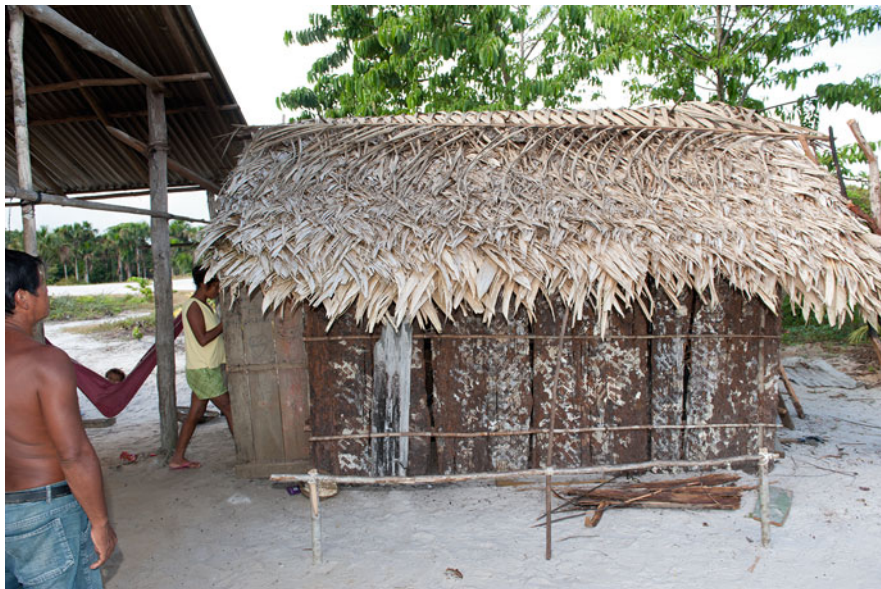
Fig. 16.2 External kitchen of a Tukano home. The roof is thatched with fronds of a Geonoma palm with an elongated frond of Attalea sagotii at the apex to help weigh down the other fronds in the event of a storm. São José, Rio Tiquié, affluent of the Uaupés, Amazonas, Brazil, 10-29-12
