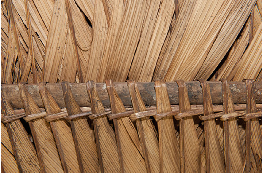
Fig. 52.7 Fronds of ubim branco ( Geonoma maxima ) attached a narrow section of the trunk ( ripa ) of bacabinha ( Oenocarpus mapora ). Roof of a manioc processing hut. Bom Socorro, Paraná Tambaqui, near Lago Amanã, Amazonas, Brazil, 9-22-12
