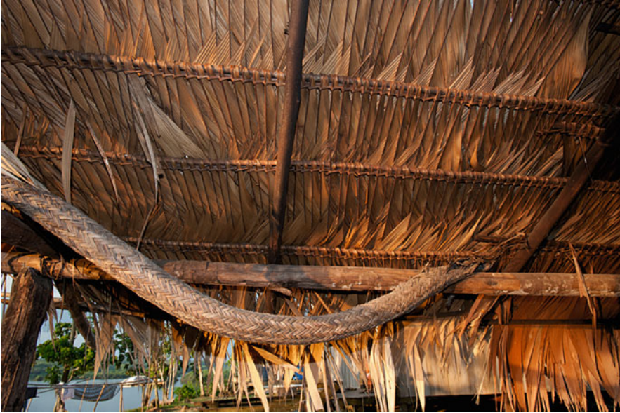
Fig. 38.5 Hut for processing manioc thatched with ubim branco ( Geonoma maxima var. chelidonura ). Smoke from the manioc oven has tinted the fronds. The sleeve-like tipití press for squeezing manioc dough hanging from the rafters is made from strips torn from the bark of jacitara ( Desmoncus polyacanthos ) palm. Ubim, Lago Amanã, Amazonas, Brazil, 9-17-12
