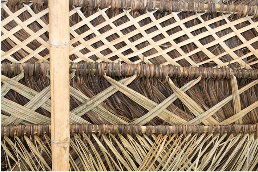
Fig. 4.5 Roof of a Kichwa house made with fronds of two palms, including Aphandra natalia , that serve as the frame for a covering of paja toquilla ( Carludovica palmata ) leaves. Canelos, Alto Pastaza, Ecuador, 9-21-13
