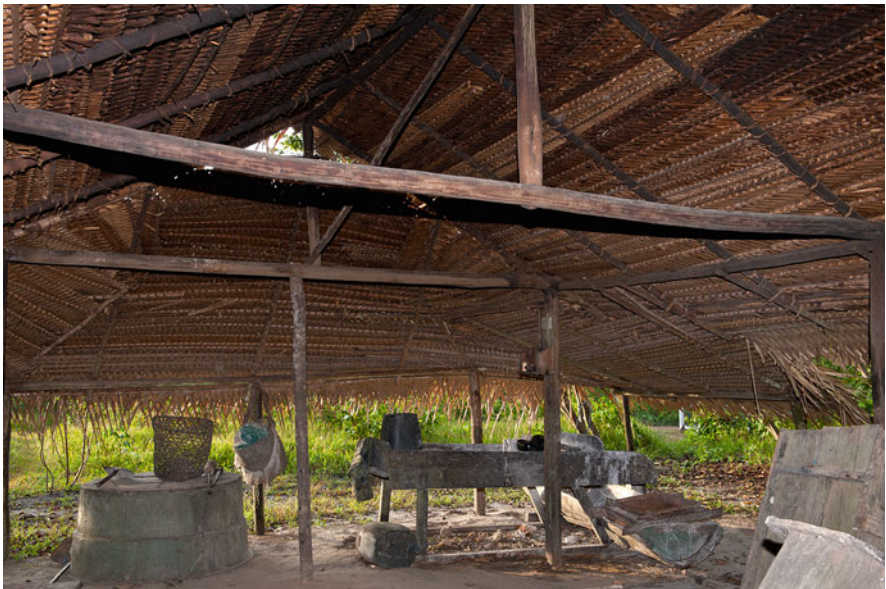
Fig. 17.10 Hut for processing manioc flour ( casa da farinha ) thatched with fronds of palha branca ( Attalea speciosa ). This 10 year-old hut has been re-thatched three times. Seringalzinho, Jaú River, Amazonas, Brazil, 10-3-12
