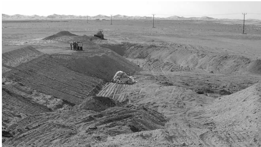
Figure 12. In January 2004 the sediments of the experimental pit were excavated, and the pit was closed starting from the northern side. The slope on the left used to be the southern bank.
