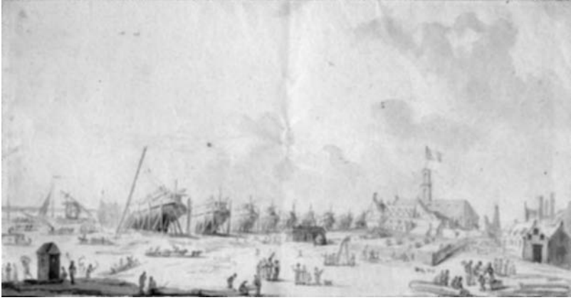
Figure 13.1 Napoleon's New Shipyards in Antwerp, artist J. van Regenmorter, water-colour, c.1804, private collection, Berchem, Belgium
