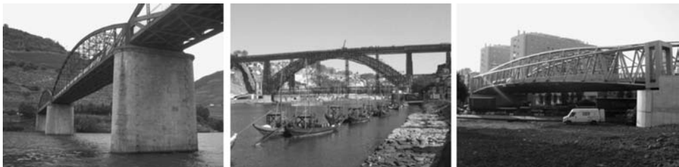
Figure 1. Structures observed with monitoring systems. Left: Pinhão bridge, northern Portugal; Center: Luiz I bridge, Porto; Right: Andreas viaduct, Porto.
