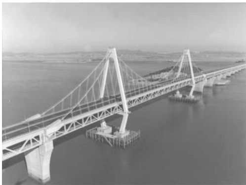
Figure 1. Overview of Yongjong Bridge.
