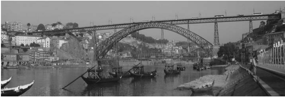
Figure 5. Overall view of Luiz I bridge.
