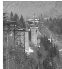
Verrand viaduct (2001). Connection of the two semi-bridges (during launching)
