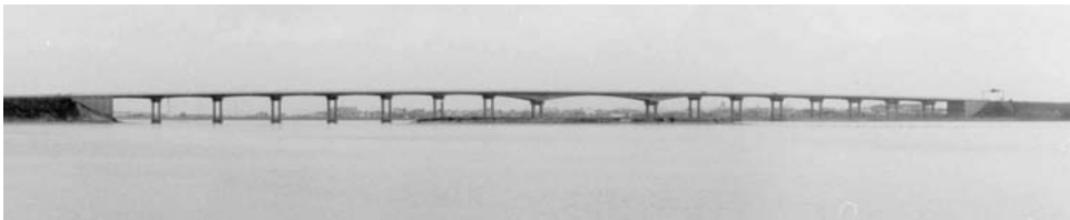
Figure 1. General view of the Barra Bridge.
