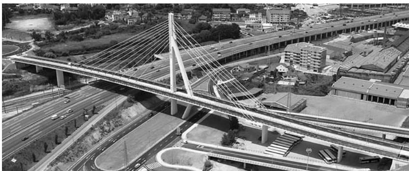
Figure 1. General view of the cable-stayed bridge (© F. Piqueiro, Foto Engenho, Lda.).
