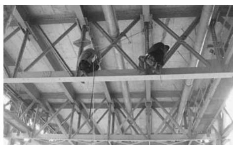
Figure 5. Installation of Strain Checker by rock climbers.
