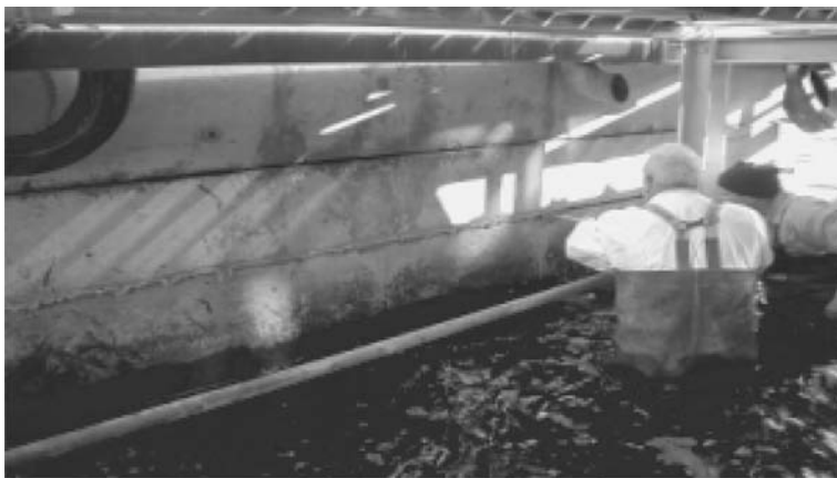
Figure 1. The Faro Bridges. Casting of slots with inserted anode ribbons. November 2001.
