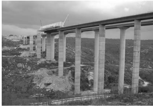
Figure 2. 100 m high C6a Bridge – Portugal – 2002
