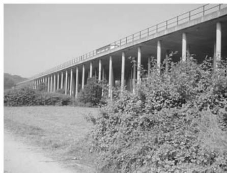
Figure 2. Partial elevation of the access viaduct.
