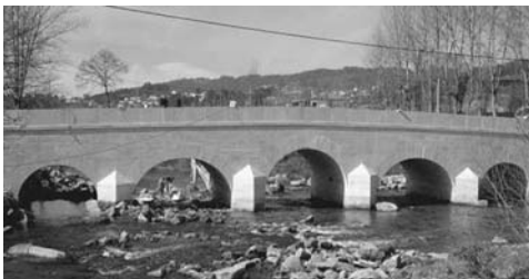
Figure 1. The Vila Fria new stone masonry bridge.
