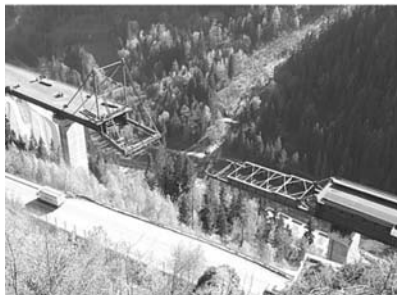
Verrand viaduct (2001). Connection of the two semi-bridges (during launching)
