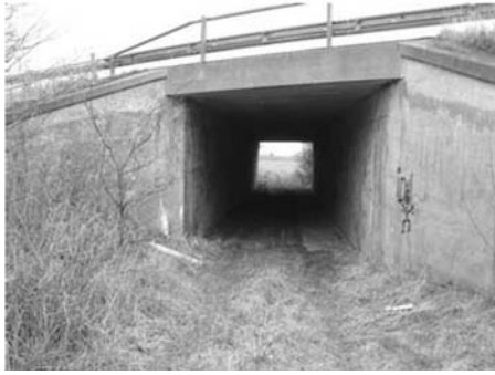
(a) Bridge at Rødbyhavn Elevation
