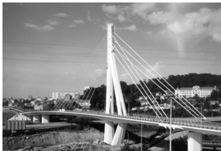
Figure 2. (a) The Viaduct over VCI in Oporto. A cable stayed bridge (central suspension) with a main span of 120 m; Fig. 2(b) Eigenfrequencies of the stays from the power spectrum.
