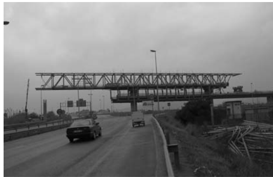
Figure 3. High speed train Bridge – Barcelona – 2005
