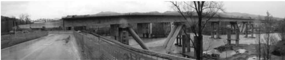
Figure 3. The Reno bridge during launching.
