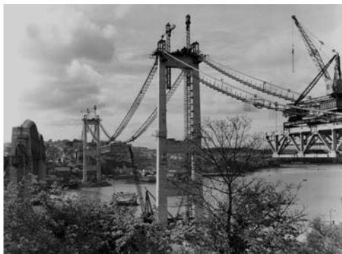
Figure 1. Tamar Bridge under construction.
