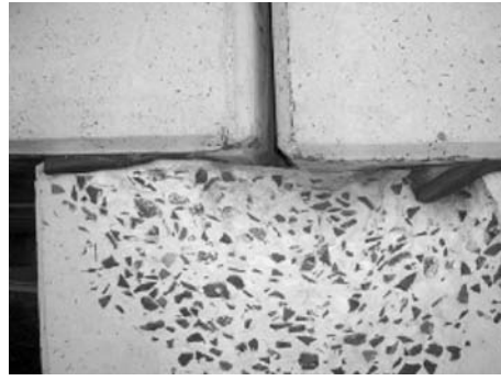
Figure 2. Displacement and contact of bearing surfaces.
