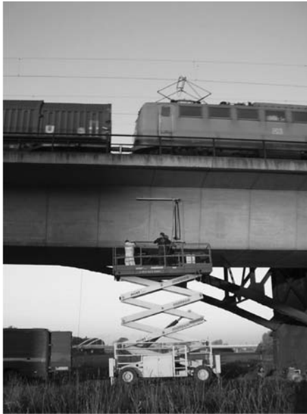
Figure 1. Scanning system at a German railway bridge.
