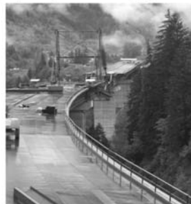
Verrand viaduct (2001). Connection of the two semi-bridges (during launching)
