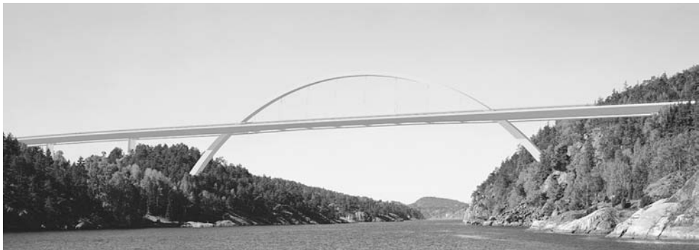
Figure 1. An artists impression of the New Svinesund Bridge, seen from east. The main span consists of a single arch carrying one bridge deck on each side (from Vägverket (2005)).
