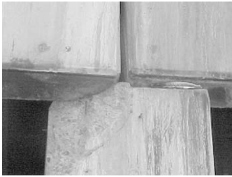
Figure 1. Spalling.
