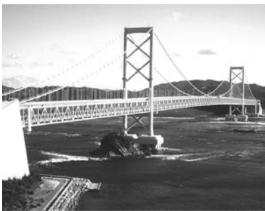
Figure 1. The Ohnaruto Bridge, completed in 1985 and repainted in 1998–2005.
