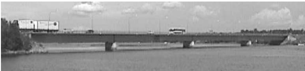
Figure 1. Elevation of the E4 Bridge over Piteå River in Northern Sweden.
