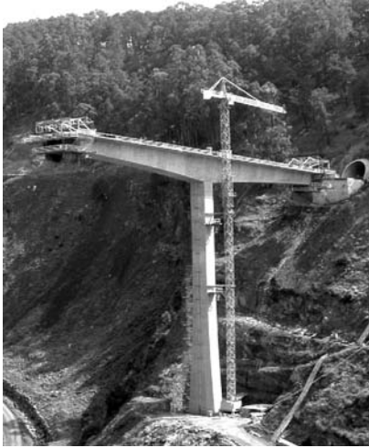
Figure 1. (a) The Ribeira Finda bridge, in Madeira Island. Main span 135 m; Fig. 1(b) Curved balanced cantilever bridge during construction.
