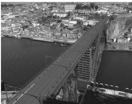
Figure 1. The Luiz I Bridge during the rehabilitation process.
