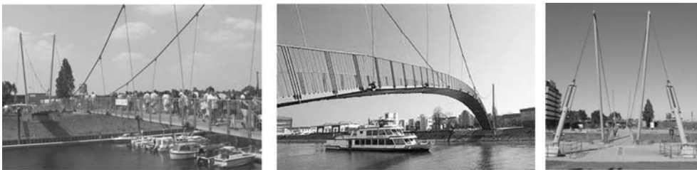
Figure 4. View of Katzbuckelbrücke in Duisburg.
