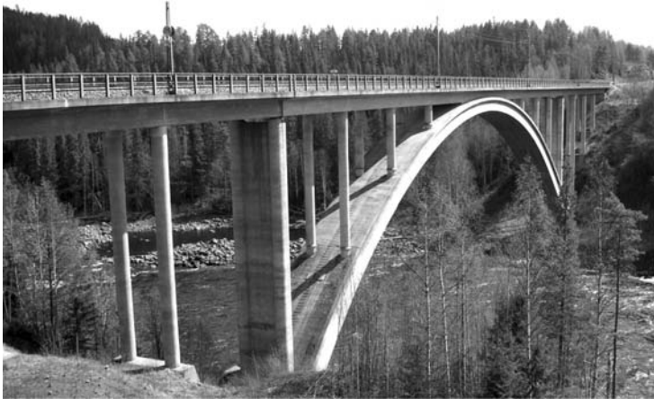
Figure 1. Bridge over the Vindel River in northern Sweden.
