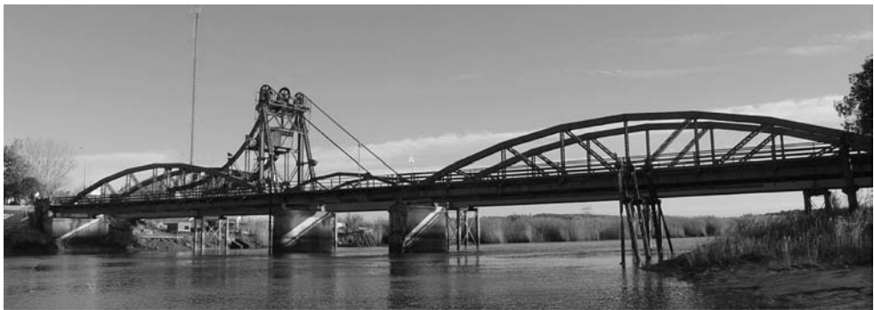
Figure 1. General view of the bridge.
