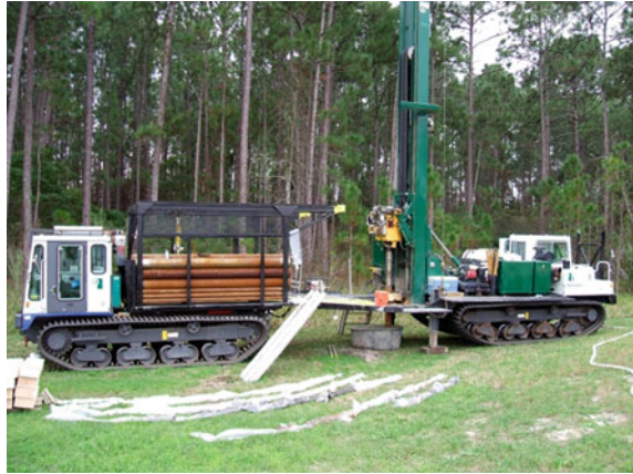
Fig. 6.9 Sonic drilling rig. Collected cores were laid out on visqueen for description and then boxed and archived
