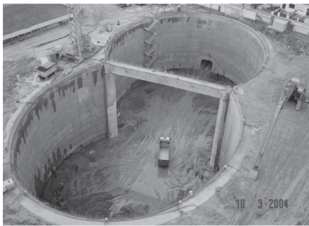
Figure 2. Final excavation phase for Salgueiros Station (Topa Gomes et al., 2008).
