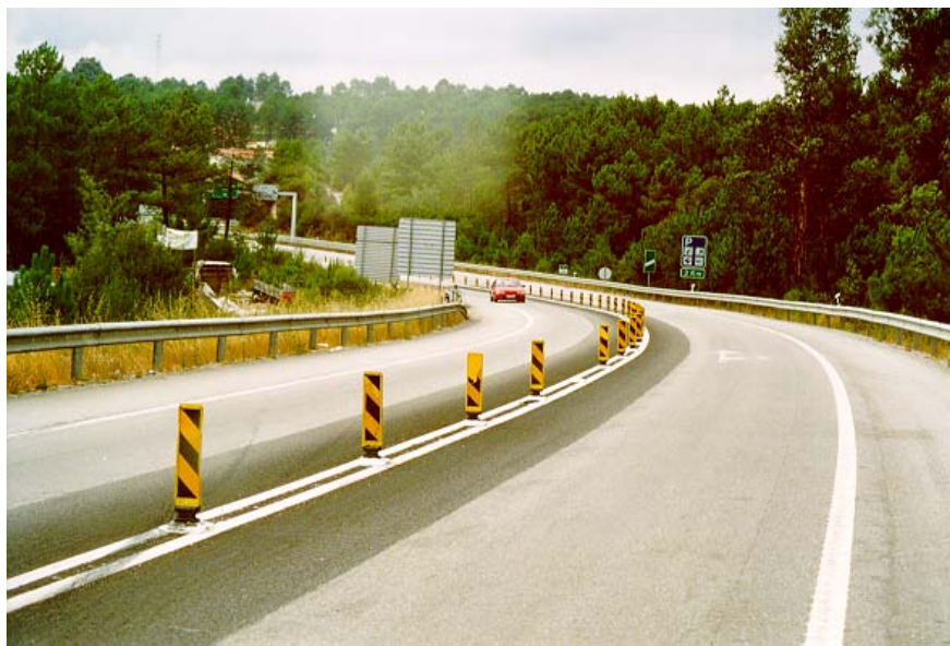
Figure 2 Position marker posts at the road axis at the approach to an interchange
