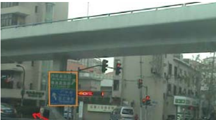
Figure 7. Turning point of the second route with irregular structure
