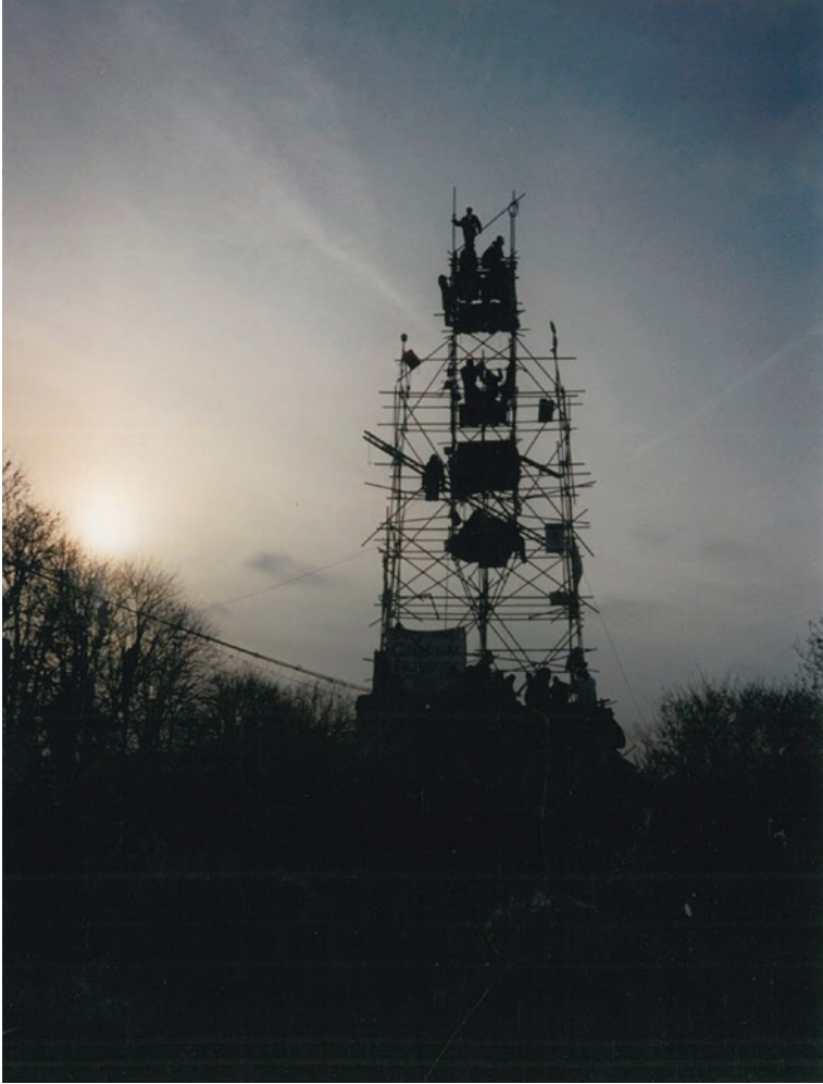
Fig. 2.12 As the eviction drew near, the inhabitants of Claremont Road erected 'Dolly's Tower' which, as in the children's story The House that Beebo Built , emerged from the top of a roof (Image by Maureen Measure, courtesy of the author)
