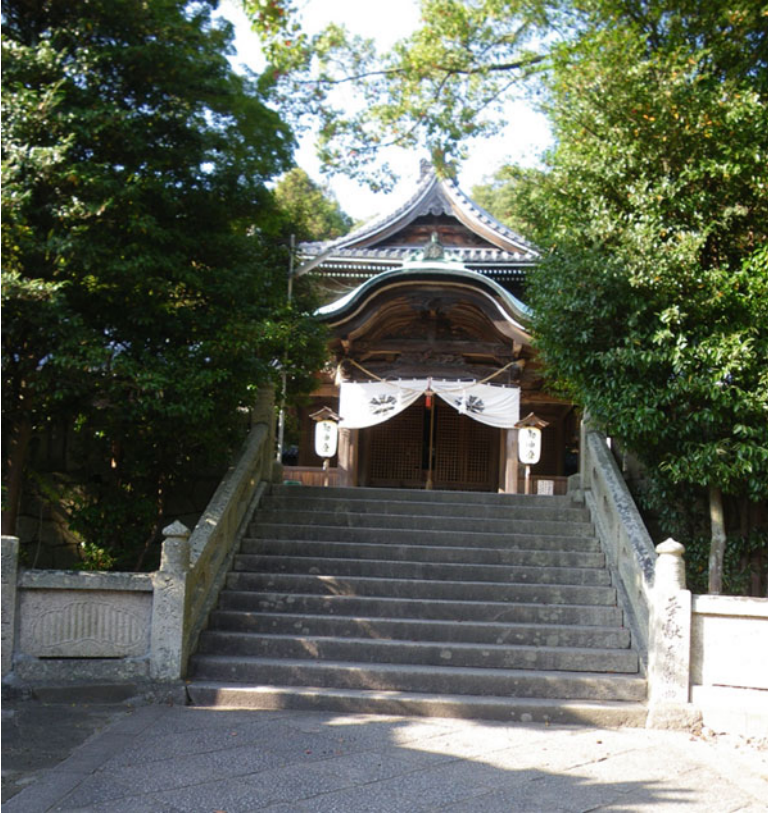
Fig. 3.43 Stone steps in front of the main building of Osake Shrine. Each step is made of one stone
