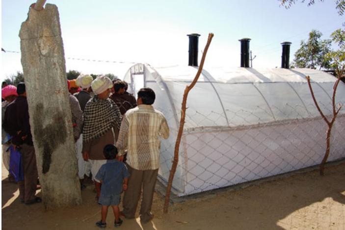
Fig. 14 Local tunnel solar drier
