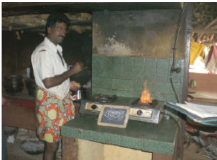
Fig. 7 Home cooking on biogas generator
