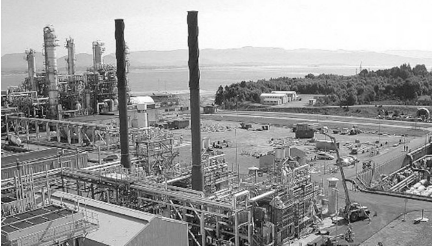
Fig. 3 Plant X, six boilers
