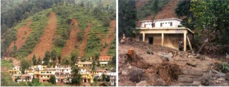
Fig. 12.7 Phata Byung Landslides on Guptkashi–Kedarnath road
