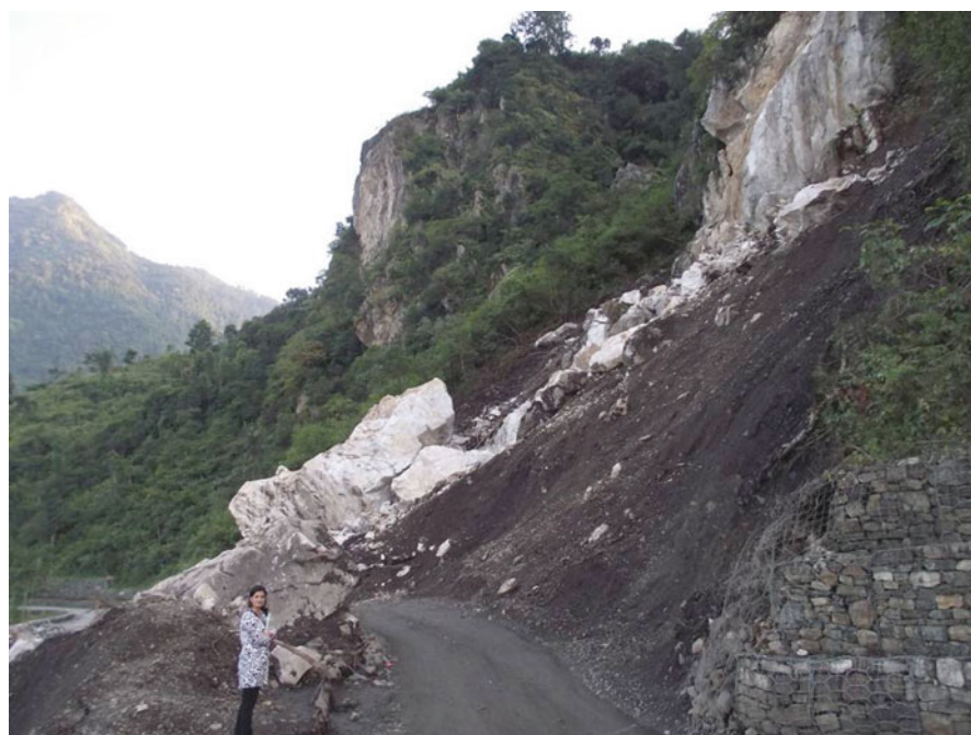
Fig. 4.3 Photographs of earthquake triggered landslide in Bhedetar along Dharan-Dhankuta road in Nepal. This landslide was triggered by Sikkim-Nepal border earthquake of 2011 (Photo courtesy: R.K. Dahal)
