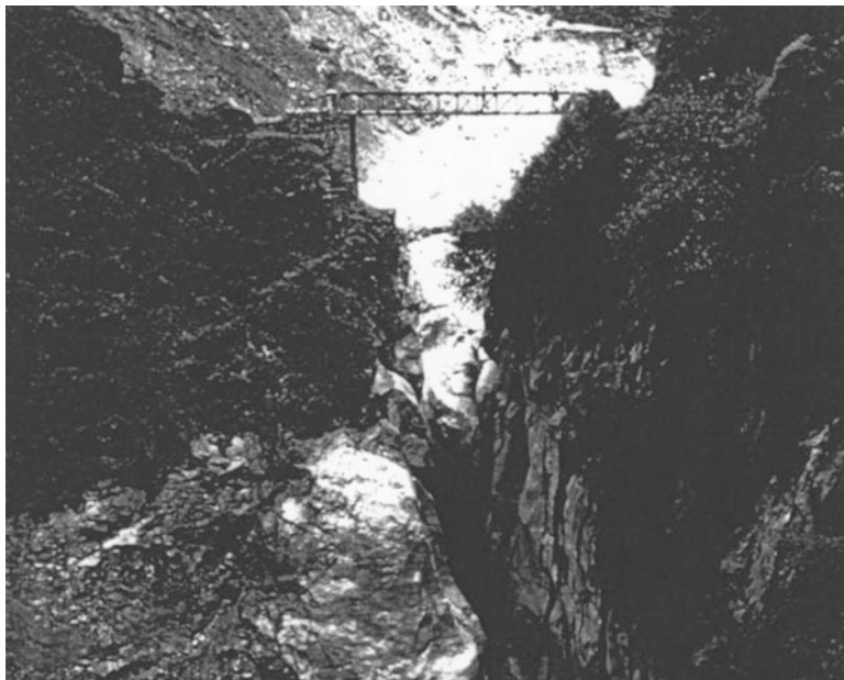
Fig. 12.4 A rare catastrophic landsliding and flooding in Alaknanda river
