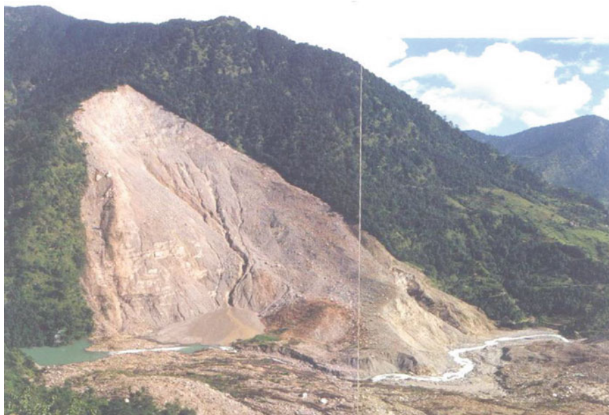
Fig. 12.6 A panoramic view of Bhenti-Paundar Landslide
