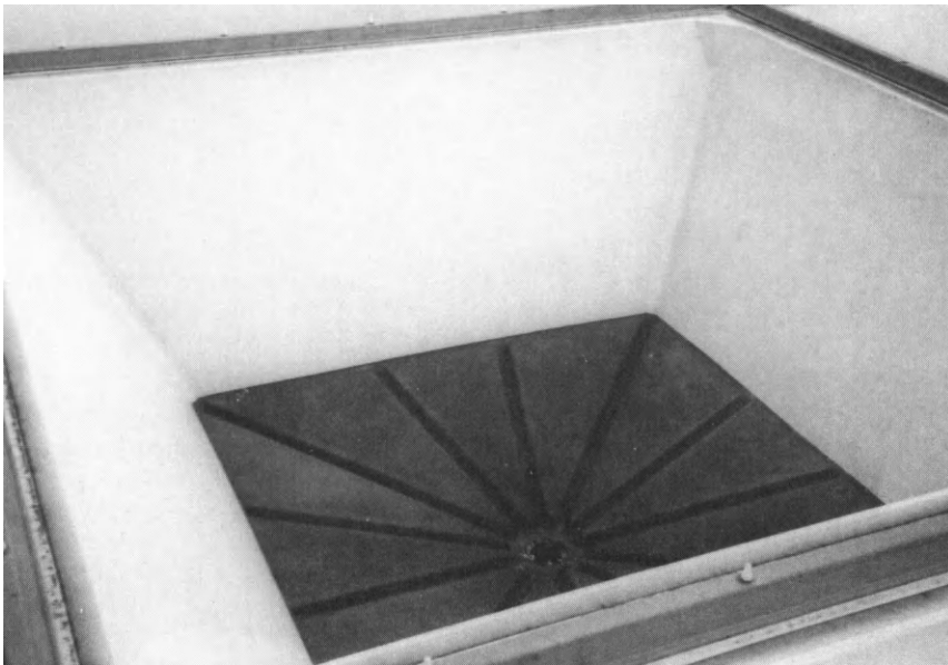
Figure 9.6 New Covent Garden roof showing individual drainage of each module
