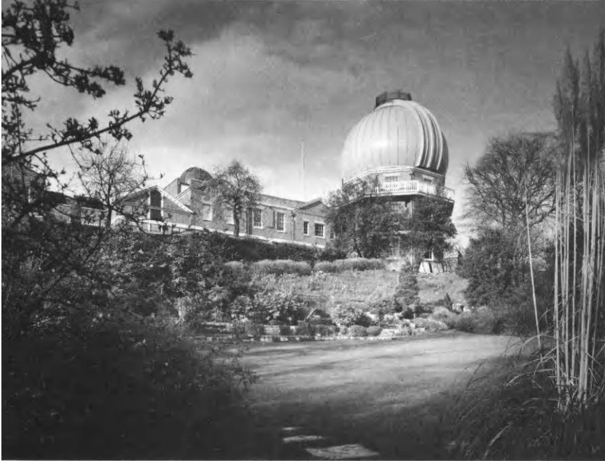
Figure 1.5 The 9 m diameter GRP dome on the Great Equatorial Building, Greenwich Observatory. The dome replaces the iron-framed papier maché original which was erected in 1895 and destroyed in the Second World War
