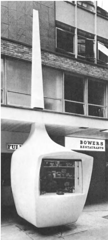
Figure 7.2 A GRP moulding exhibiting two dimensional curvature and 'saddle' curvature. Such units would be extremely rigid in themselves
