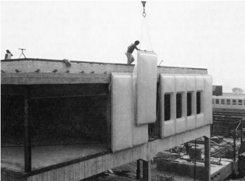
Figure 7.3 Dishing, albeit shallow, of these panels imparts considerable natural rigidity
