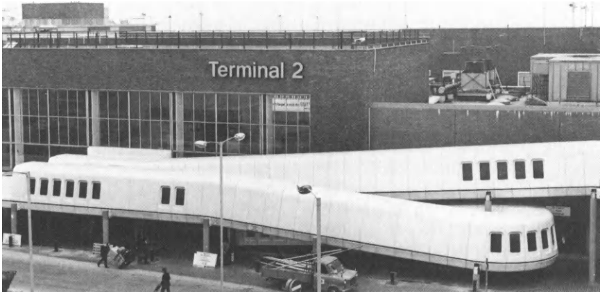
Figure 10.6 GRP access ramps at Heathrow Airport
