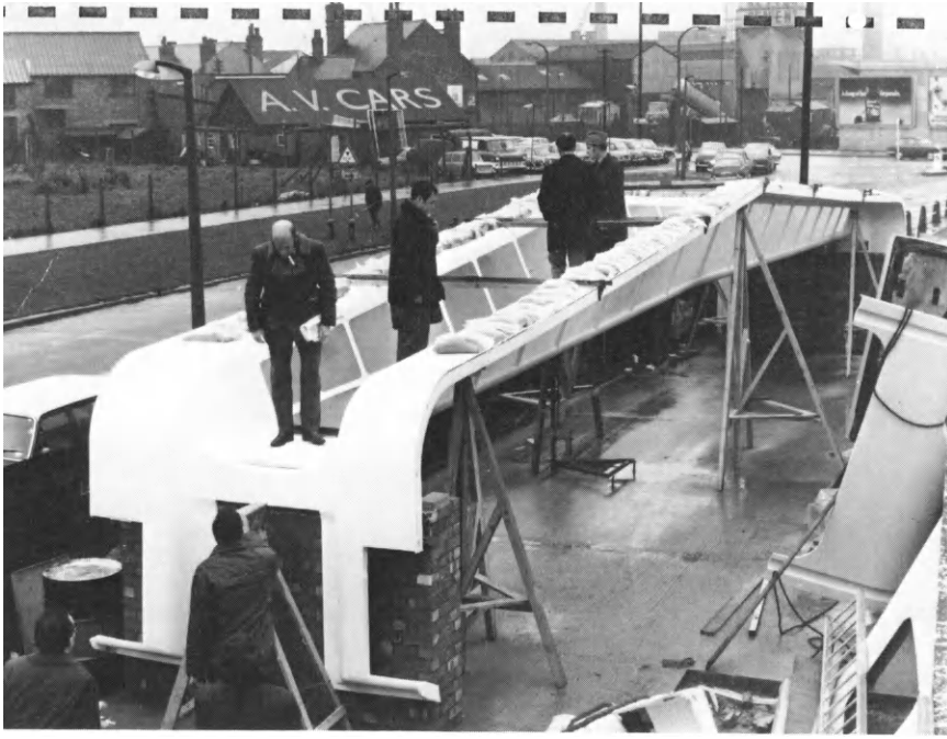
Figure 8.13 Full-scale load test on roof for Morpeth School, London
