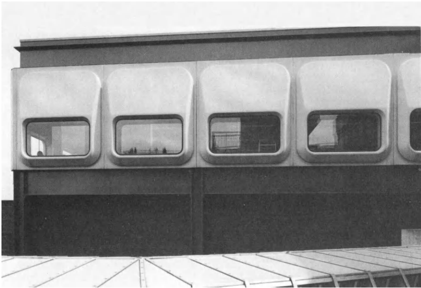
Figure 7.8 The panels at Heathrow Airport. Although not extreme examples, the picture illustrates the effect of clearly defined light and shade areas
