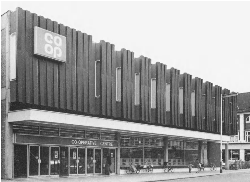
Figure 3.5 A store in Bedford. Bold and innovative use of GRP. Clearly the design does not relate to any other building material
