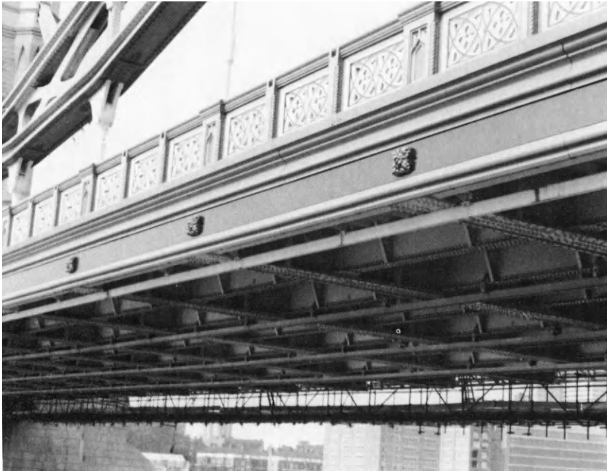
Figure 1.3 GRP mouldings replacing cast iron decorative work on Tower Bridge, London
