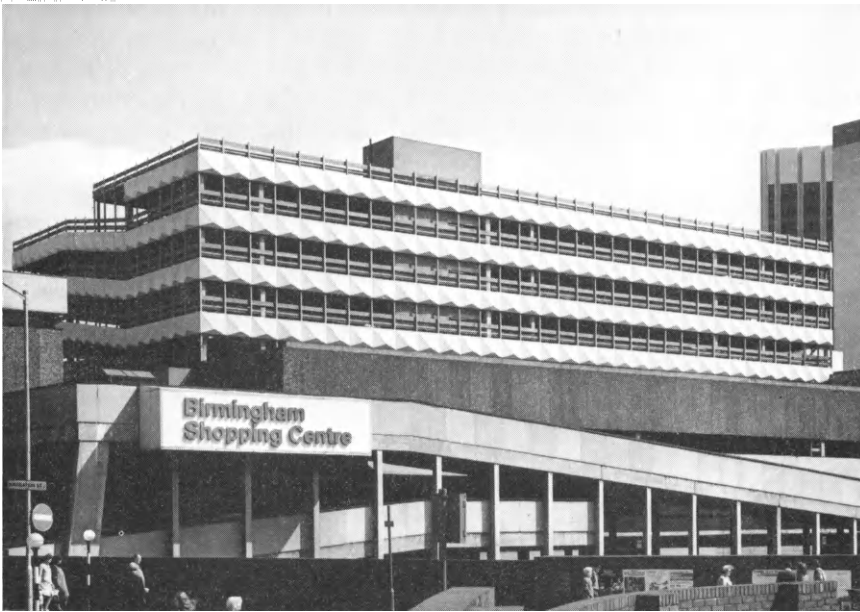
Figure 3.4 GRP cladding to multi-storey car park. The uniformity of shape, colour, texture and weathering gives clarity and meaning to repetition of a simple geometry
