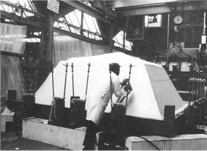
Figure 5.8 Assembling reinforcement and insulation slabs on to male mould
