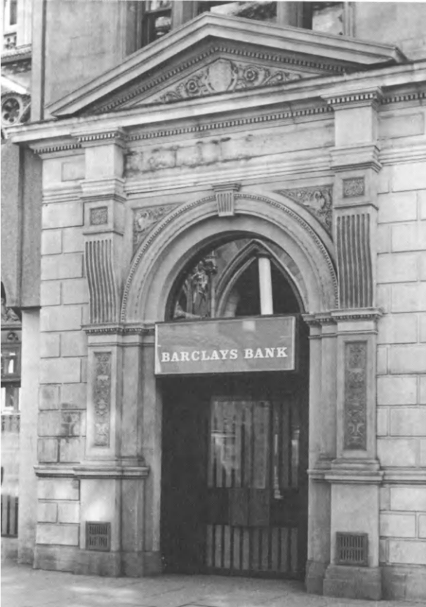
Figure 1.4 The arch and doorway is moulded in GRP, the mould has been taken directly from the original masonry which exists at the other end of the same building
