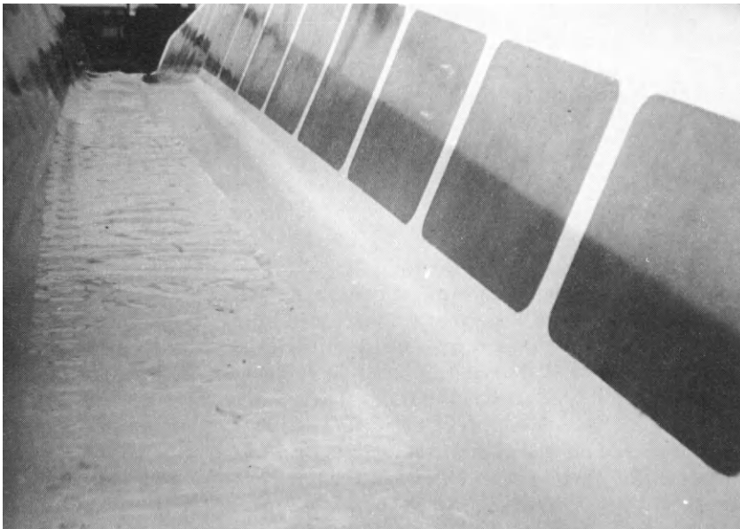
Figure 7.1 GRP roof unit incorporating rain water run-off and, through translucent panels on right, natural lighting (Morpeh School, London)
