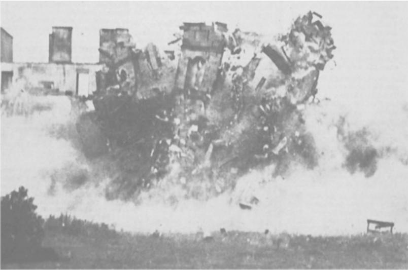
**FIGURE 1** *Demolition of Rosneath Castle, Argyll and Bute, in 1961, by 220lbs of gelignite*
