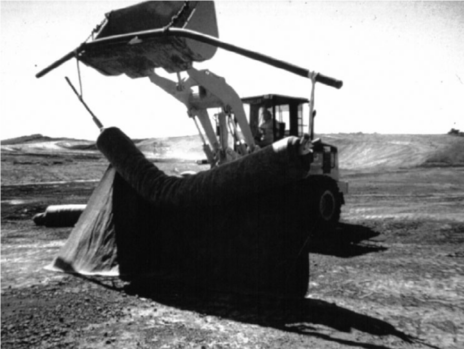
Figure 5-6. An Unacceptable Situation for Field Deployment of a GCL.
