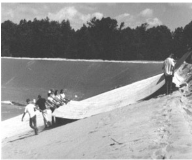
(c) Field deployment of a GCL by stationary roll pull method
