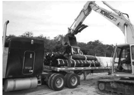
(b) GCLs Being Unloaded Using Dedicated Slings
