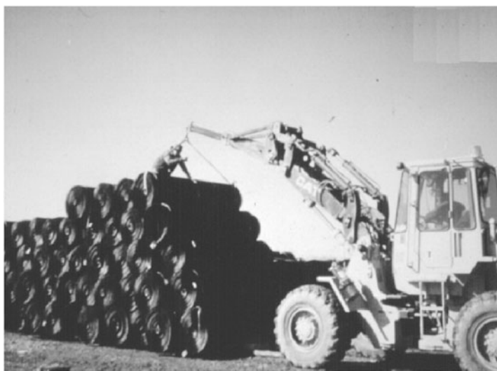
Figure 7-10. Geonets Being Temporarily Stored at the Job Site.
