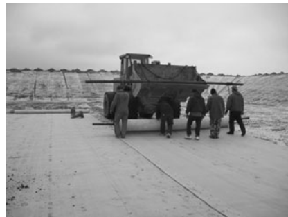
(d) Field Deployment of GCL on Soil Subgrade with Controlled Overlap
