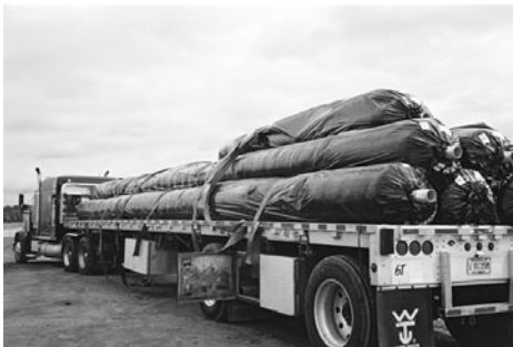
(a) GCL Being Delivered to the Job Site
