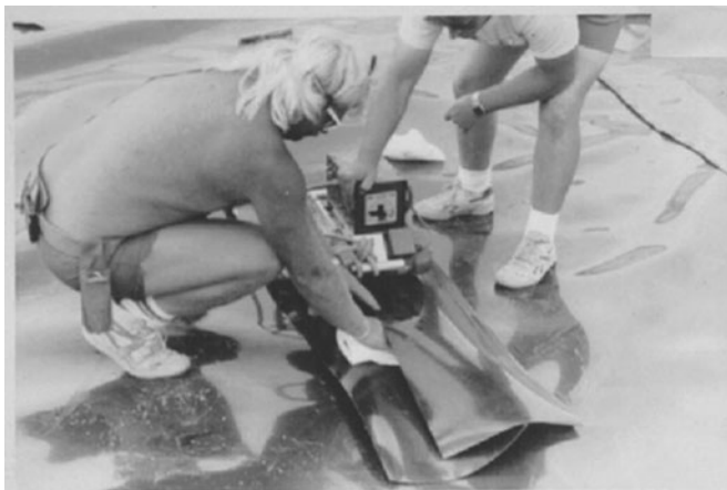
Figure 4-20. Fabrication of a Geomembrane Trial Seam.
