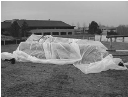
(c) Temporary Storage of GCLs at Job Site
