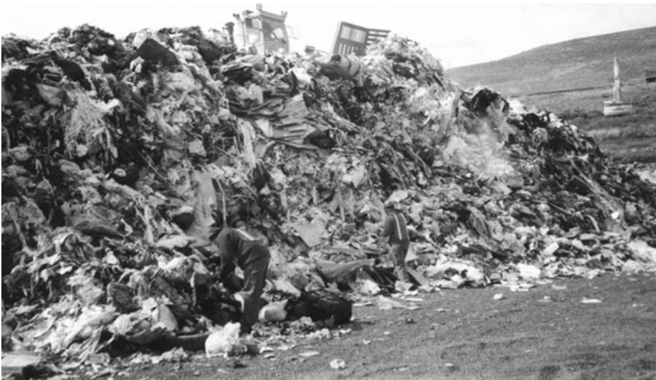
Figure 6-4. CQC and CQA Personnel Observing Placement of Select Waste on a Drainage Layer.
