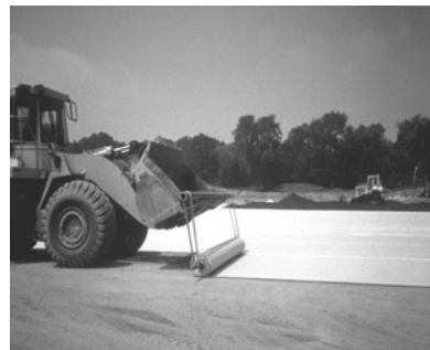
(d) Field deployment of a GCL by moving roll pull method
