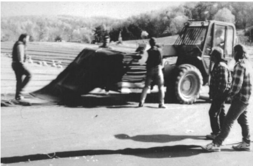
Figure 4-15. Photographs Showing the Unrolling (upper) and Unfolding (lower) of Geomembranes.
