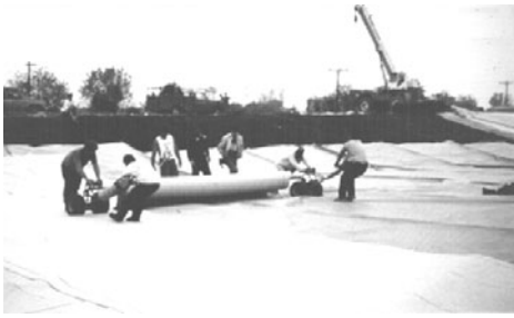
(a) Field deployment of a GCL by manual unroll method
