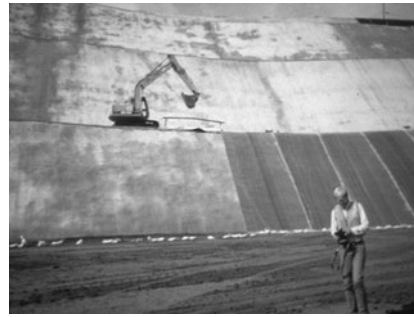
(b) Field deployment of a GCL by gravity roll release method
