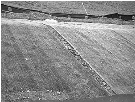
(c) Separation of GCL panels \approx 300 mm (12 in.)
