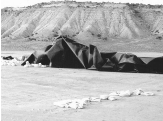
Figure 4-17. Wind Damage to Deployed Geomembrane.
