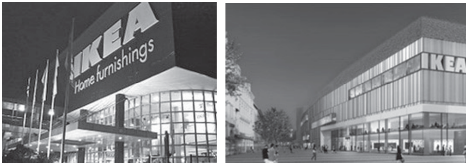
Figure 3.5 Examples of IKEA City Stores (in Queenstown, Singapore (left), and in Hamburg, Germany (right))
