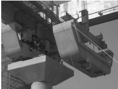
Fig.9 Pier segment lifting (simple span)
