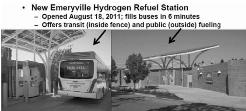
Figure 2 AC Transit Emeryville Refuel Station Dispensing Locations
