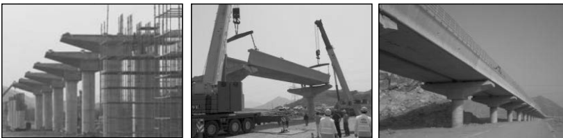
Figure 4. Erection stages on the line
