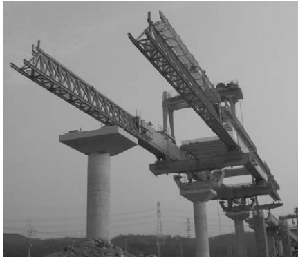
Fig.10 Launching girder during positioning stage
