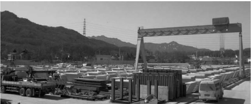
Fig. 8 Casting yard overall view with gantry crane line 1
