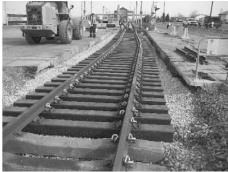
Figure 3: Installed Axion International plastic composite ties using traditional wood equipment.
