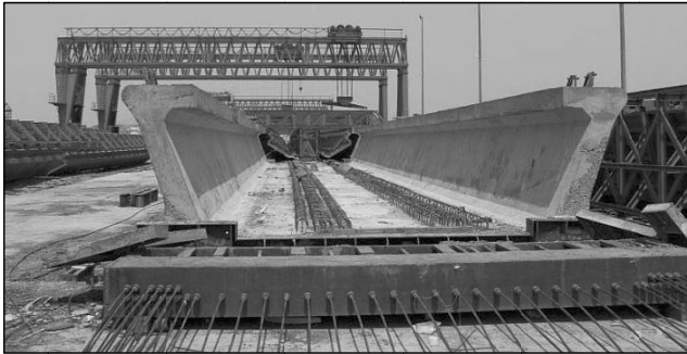
Figure 3. Prefabrication of typical viaduct
