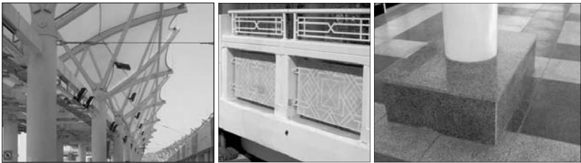
Figure 9. Canopy, guardrails and tiling
