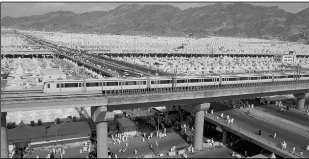
Figure 5. King Abdullah Overpass (27-45-27m) in operation double track, constant depth, balanced cantilever method
