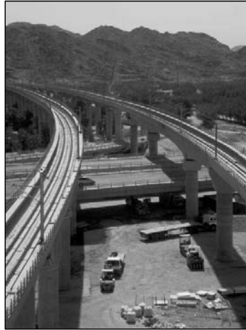
Figure 7. Twin King Faisal Overpasses (35-58-35m) single track, variable depth, curved, balanced cantilever method
