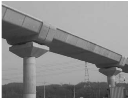
Fig. 11 Typical simple span erection completed
