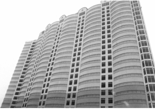
Figure 14. Wind engineered storm shutters protected this condominium building from hurricane Wilma (Courtesy of Steven Camposano).
