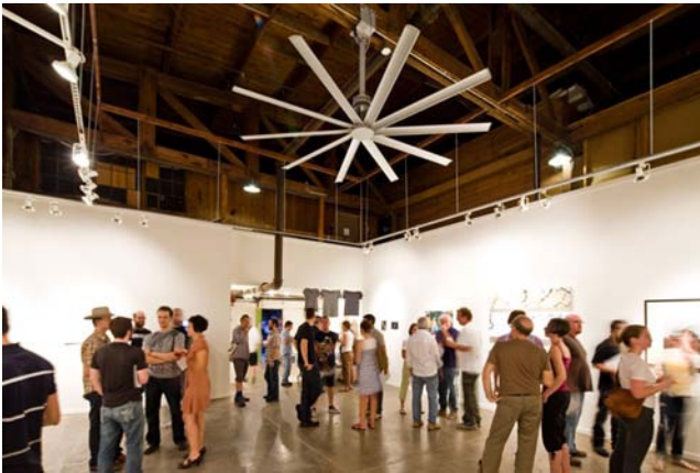
Figure 28. High-Volume Low-Speed Energy-Efficient Ceiling Fans (Courtesy of Big Ass Fan Co.).
