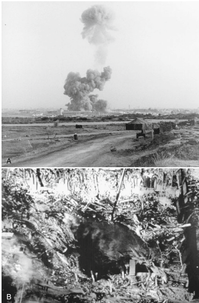
FIGURE 16.5. (A) Blast of the suicide truck bombing of the four-story U.S. Marine barracks at Beirut, Lebanon, international airport, October 23, 1983, using an ammonium nitrate-based bomb constructed as a fuel-air explosive, from 1 mile away. (B) The resulting complete building collapse with over 350 men inside.
