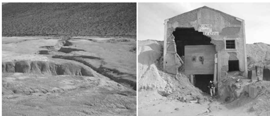
Fig. 10.1 Pan de Azúcar mine. View of the tailings ( left ). Grinding plant ( right )
