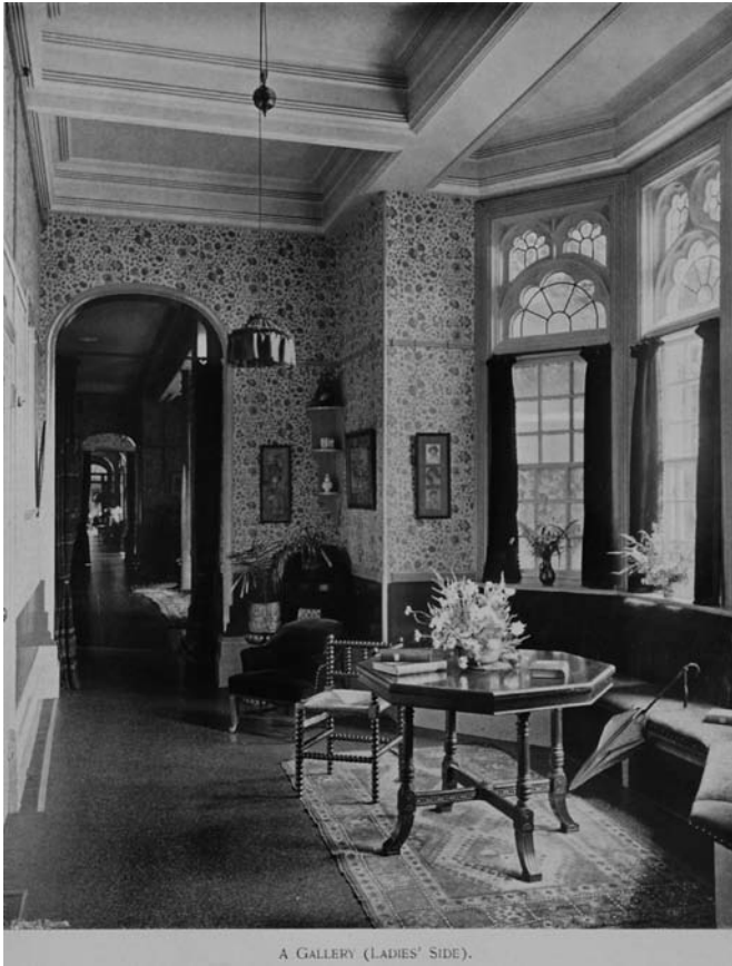
Figure 2.2 The corridor form of the female gallery at Holloway Sanatorium has been effectively disguised in this photograph
