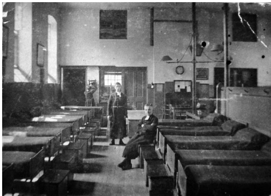
Figure 3.6 This Ward at Christ’s Hospital is typical of the ‘open dormitory’, the only personal spaces for the boys were the boxes at the ends of the beds
