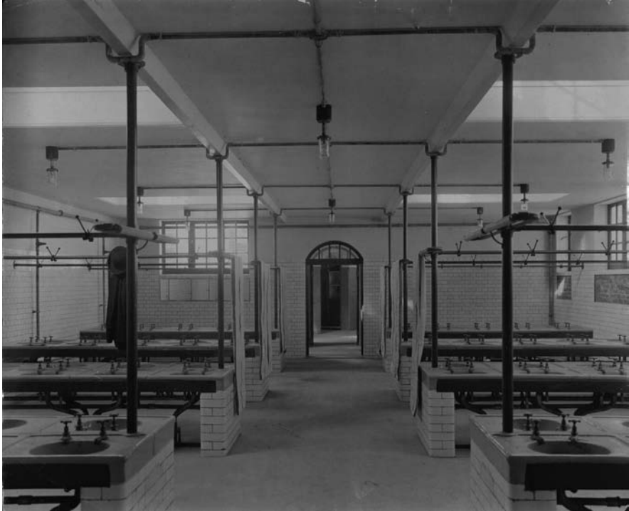
Figure 6.6 The lavatories at the London County Council's Carrington House are typical of the increased emphasis on washing facilities
