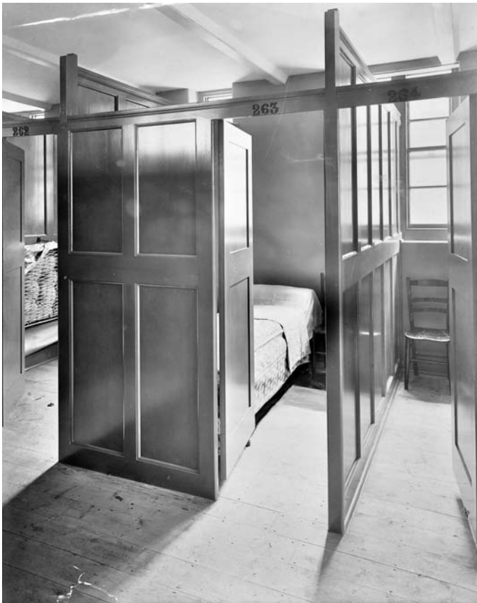
Figure 6.4 Cubicles at the London County Council's Bruce House
