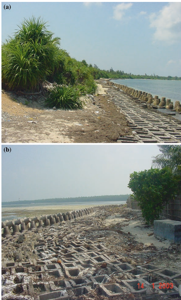
Fig. 3.16 a Hollow concrete blocks and tetrapods protecting the coast of Minicoy Island. b Another view of hollow concrete blocks and tetrapods placed on the slope
