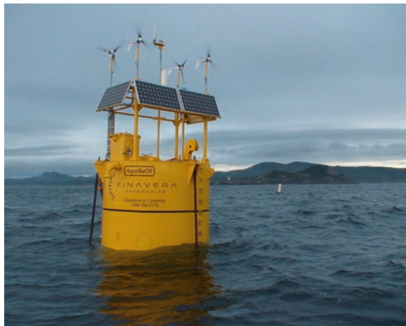
Fig. 5.5 A multi-source (wind-solar-wave) power generator system. Source http://www.finavera.com/
