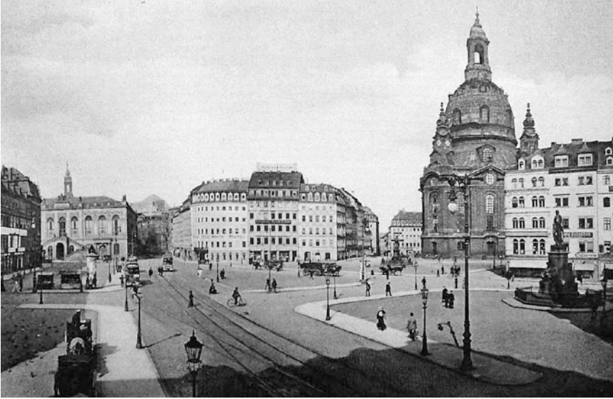
Figure 14.2 George Bähr, Church of Our Lady (Frauenkirche), Dresden, in 1910; originally constructed 1726–1743.
