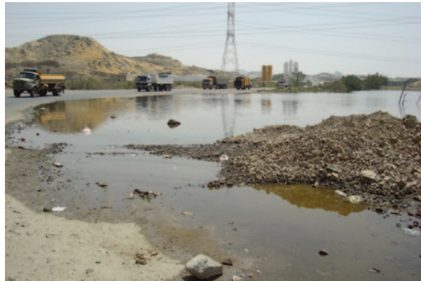
Fig. 4.7 Water accumulation along Briman road
