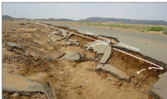
Fig. 11.3 Lateral etching of terrain materials along roads due to the lack of protection works
