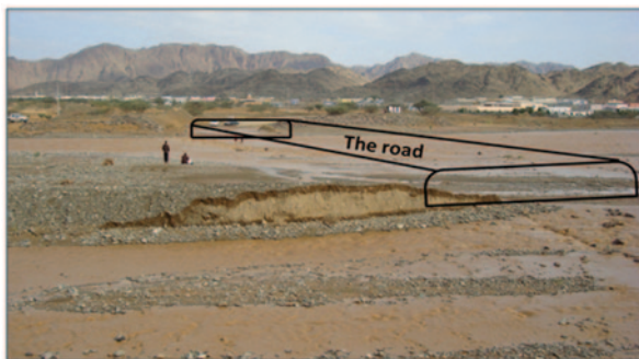
Fig. 11.11 Road cut by torrents, and a scheme of a proposed bridge
