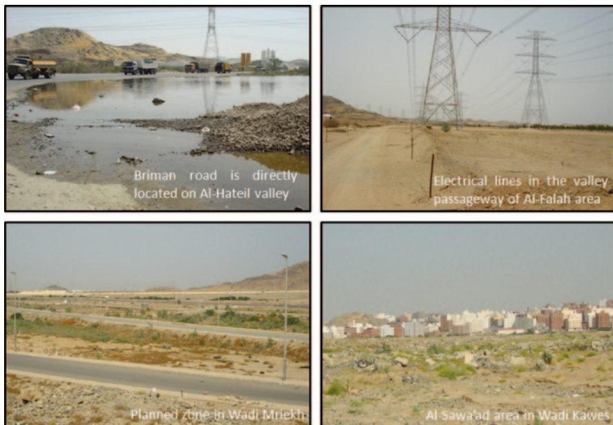
Fig. 7.6 Examples from Jeddah area showing different aspects of urban expansion in valley courses
