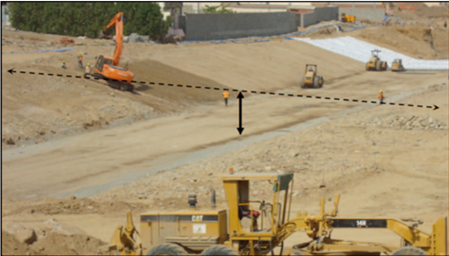
Fig. 10.14 The convey channel and the cross-section of Es-Samer Dam
