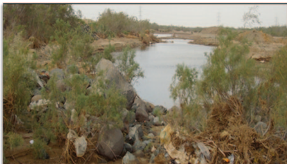
Fig. 10.5 Closing valleys passageway by rock debris near Briman road
