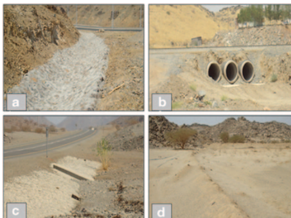
Fig. 10.2 Examples on small-scale flood controls. a Small-scale drains. b Pipes for water tunneling. c Cement tunnel. d Al-Aakoom (soil embankment)
