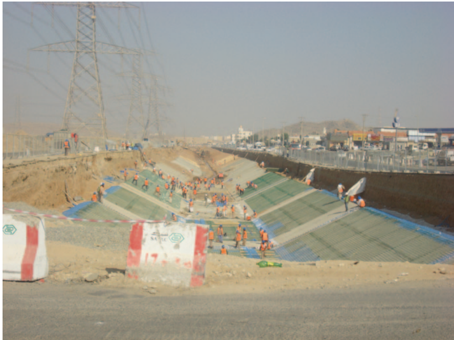
Fig. 11.14 Implementations on widening the old storm-water channel in Jeddah
