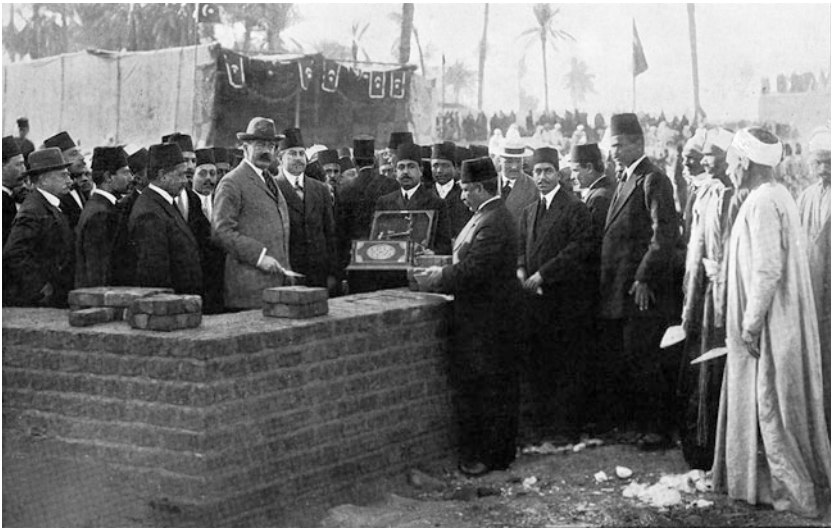
12. Kitchener laying the foundation stone of an Agricultural College near Luxor (Mary Evans)
