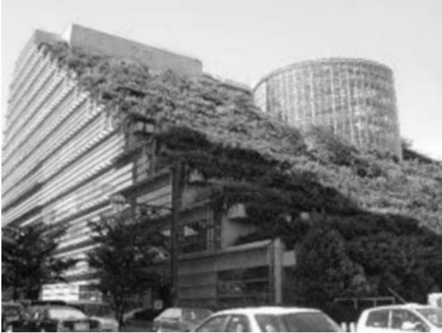
Fig. 14.25 Green building design illustrating several of the different principles of green building such as passive solar, plants for shading, etc.
