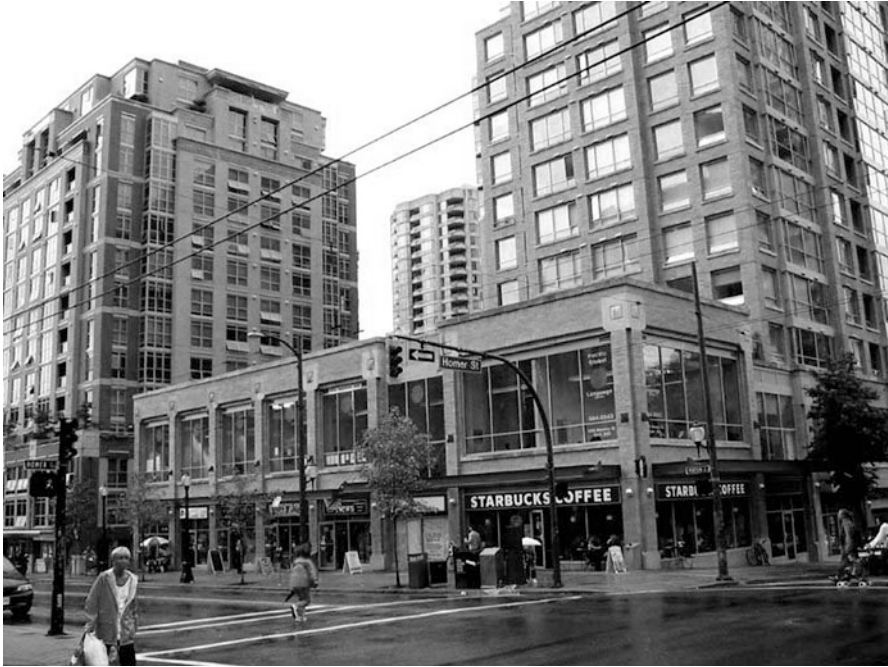
Fig. 15.1 A depiction of a section of the Southeast False Creek (SEFC) mixed-use development project in Vancouver, British Columbia, Canada
