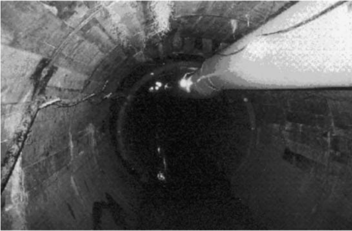
FIGURE 1.11 Inside view of a utility tunneling operations.
