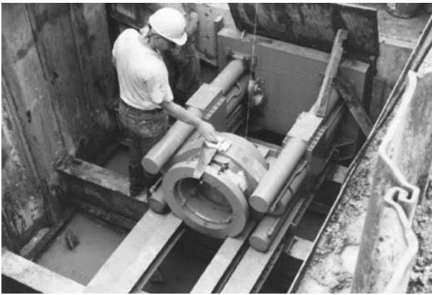
FIGURE 8.3 Jacking shaft.
