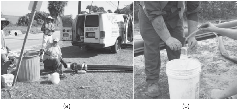
FIGURE 6.9 (a) Prechlorination and (b) sampling. (Source: Murphy Pipelines and Hammer Head.)
