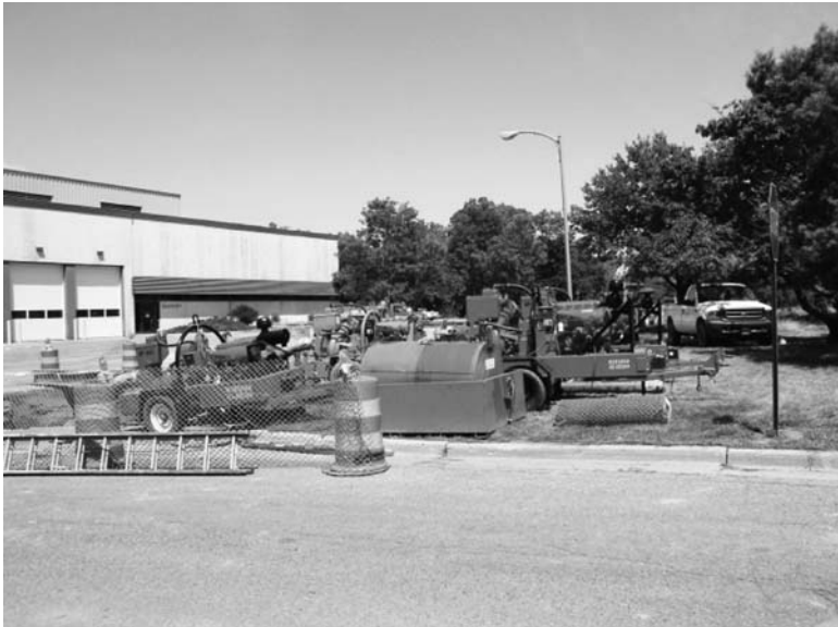
FIGURE 7.7 Typical bypass pump setup for a large volume of existing flow.
