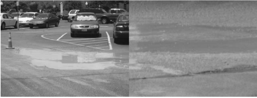
FIGURE 5.10 Inadvertent fluid returns in the urban environment.
