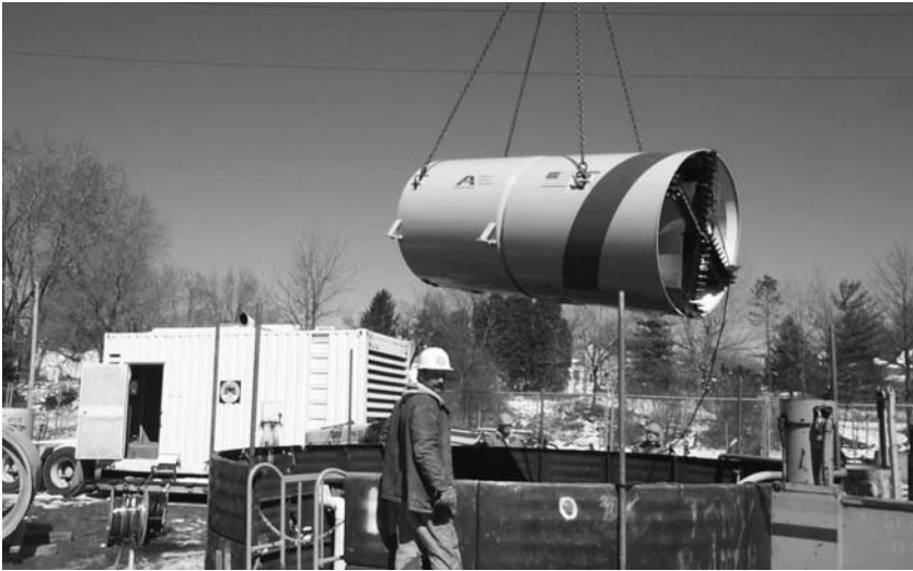
FIGURE 8.1 Conventional pipe jacking. (Source: Akkerman, Inc.)
