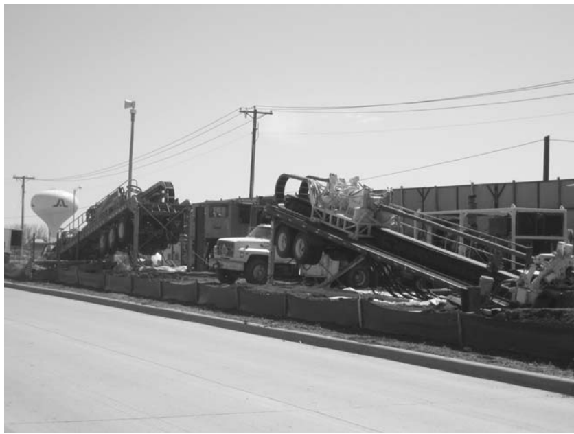
FIGURE 9.1 Staging HDD equipment to minimize environmental impacts.
