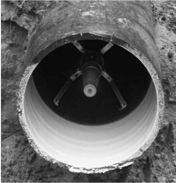
FIGURE 3.10 Polyurea lining spray head. (Source: 3M Water Infrastructure.)
