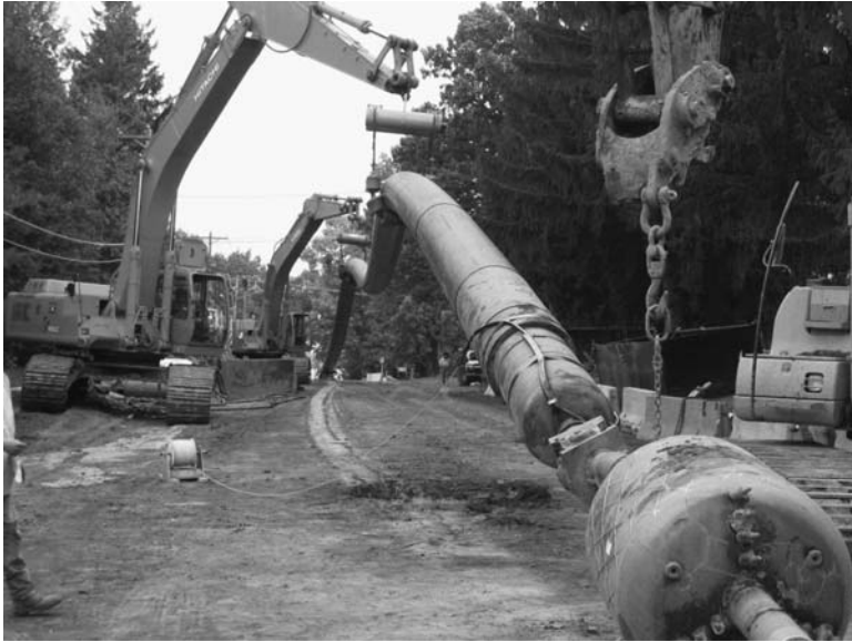
FIGURE 4.29 HDPE pipe readied for pullback in a directional bore.
