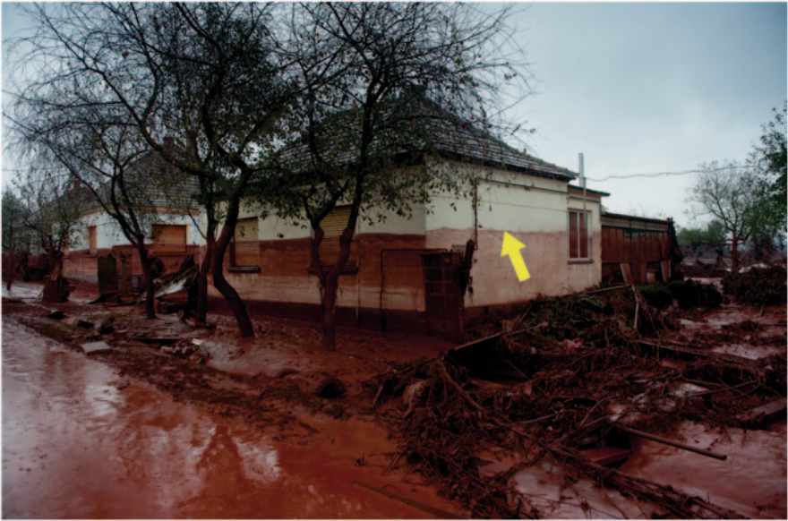
Fig. 4.15 The area around Kolontár closed by police—this was the place hardest hit by the mud wave. The arrow shows the height of the sludge level. (Picture by Ákos Stiller, permission obtained from copyright-owner)
