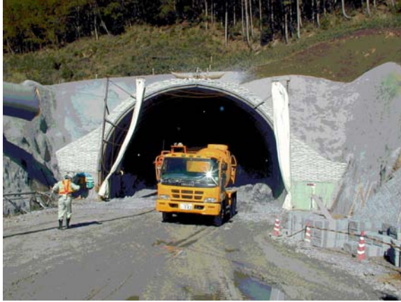
Figure 7: Suemune tunnel in Okayama, Japan.
