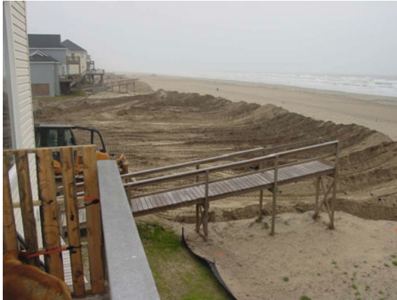
Fig. 6.4 Digging out the swale and reconstructing the foredunes, Sandhill Shores project. The reconstructed locations of the dune, swale, and their heights/depths were marked on flags for the bulldozer operator to follow. The dune was reconstructed after the storm with the aid of a GIS, GPS, and survey equipment, but the dimensions and volume were defined to match pre-storm topography, as based upon a LIDAR elevation dataset and aerial photography taken before the storm. Photo by Paul White
