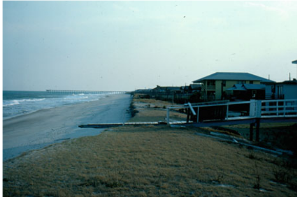
Fig. 2.2 Dune at Carolina Beach, NC, USA (1981), created using artificial fill reshaped by bulldozers into a dune-dike
