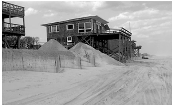
Fig. 3.8 Dune rehabilitation of the foredune positioned under the first row of houses. Sand is intermittently placed on the foredune, fences are erected, and various methods are applied to retain the sand ridge in place, Davis Park
