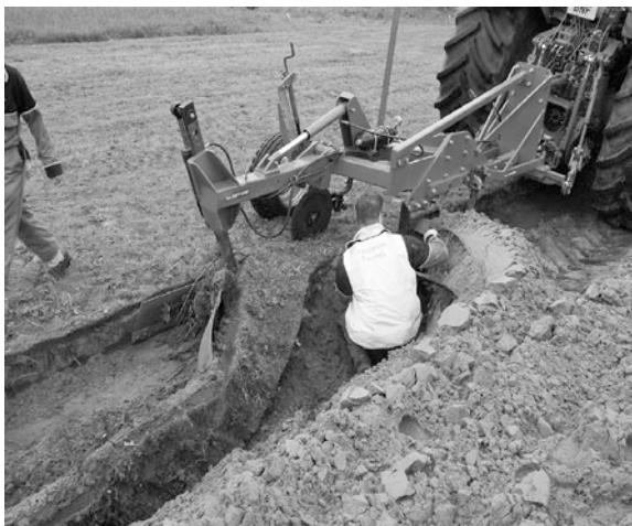
Fig. 8.5 Deep ploughing operation at Talacre Warren dune system in North Wales
