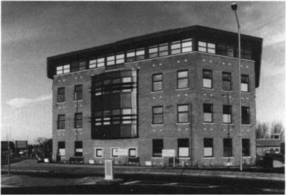
Figure 3 South west elevation of Anglia Polytechnic University Learning Resource Centre. Note the windows are divided into lower vision and upper daylighting parts with trickle ventilation wall openings below.
