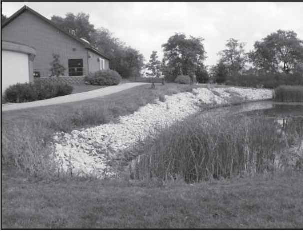
Figure 2-13 A 4,500-gpm groundwater treatment plant in Batavia, Illinois, that uses manganese dioxide filters and on-site chlorine generation to remove iron and manganese
