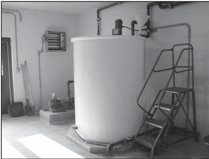
Figure 4-2 Phosphate-based corrosion inhibitors can be mixed in solution tanks from dry product or directly fed as a liquid
