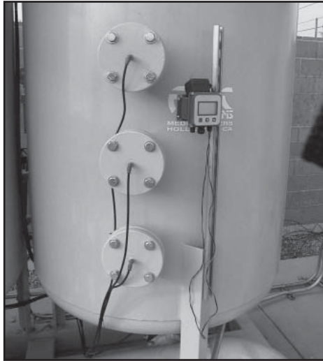
Figure 2-15 Multiple sample ports on adsorptive media vessels help track progression of contaminants through the media bed
