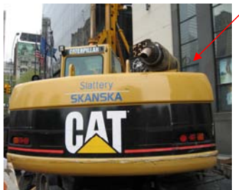
Figure 2. Excavator with DPF
